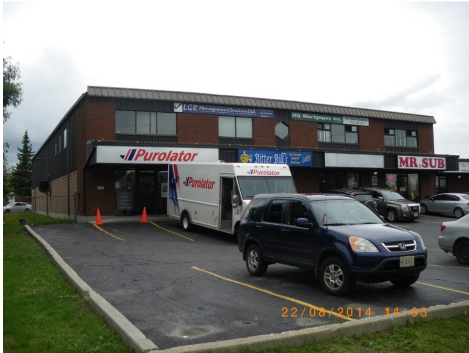
PHOTO 1 SUBJECT LANDS 1210 & 1212 LASALLE BLVD., SUDBURY VIEWED LOOKING NORTHEAST FROM LASALLE BLVD
