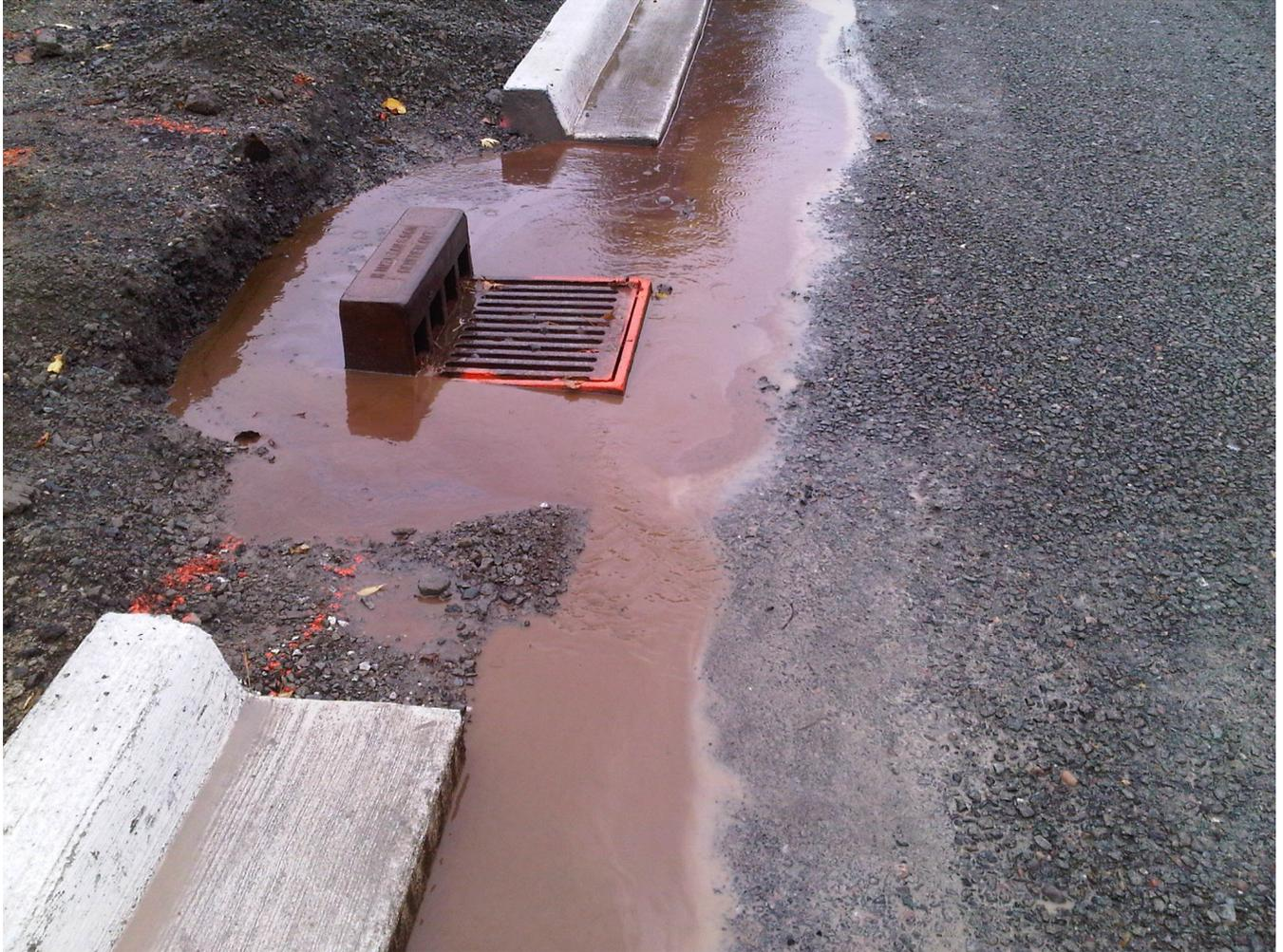
*Contaminated water entering the storm sewer system*
