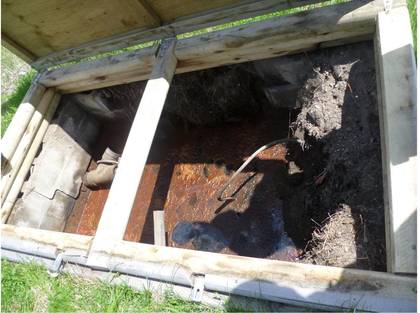
*Damaged oil interceptor requiring repair / replacement*
