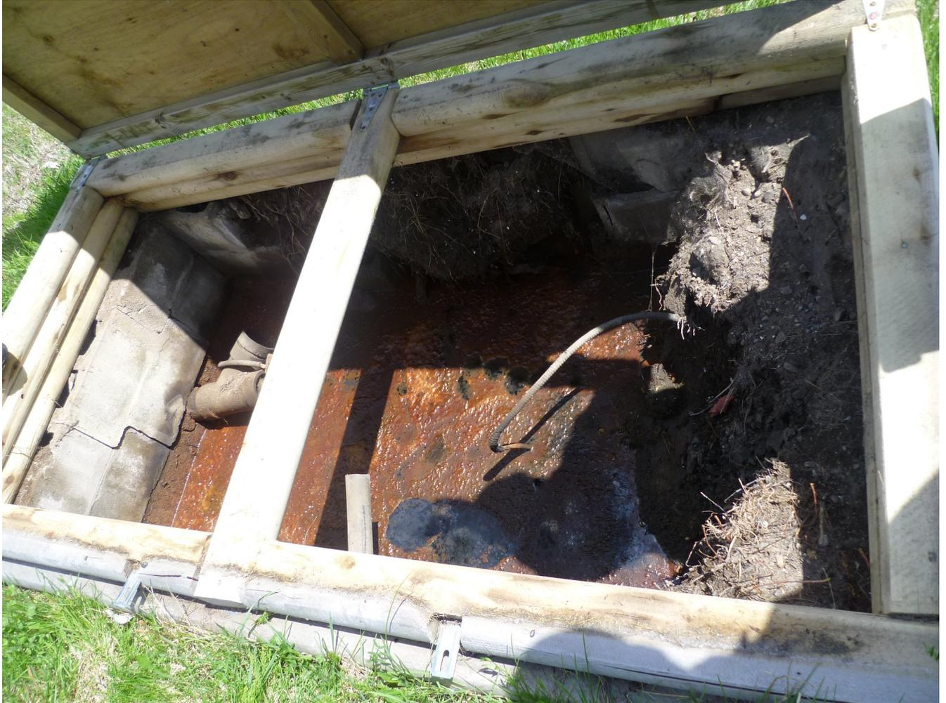
*Damaged oil interceptor requiring repair / replacement*
