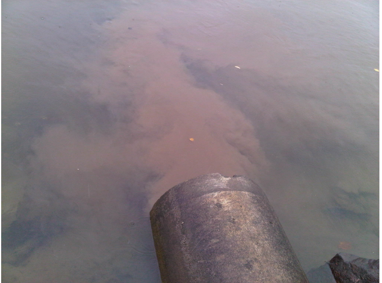
Contaminated water entering Ramsey Lake via storm sewer system
