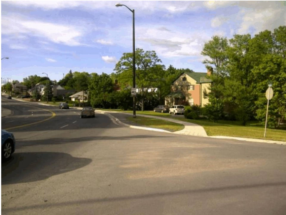
Photo 4 FROM PARIS/FACER STREET INTERSECTION LOOKING NORTH
