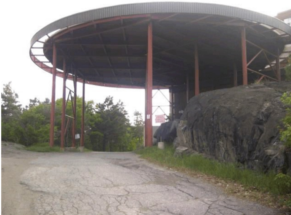
Photo 6 FROM DRIVEWAY ON/ADJACENT TO BELL PARK LOOKING SOUTH AT FORMER HELIPAD
