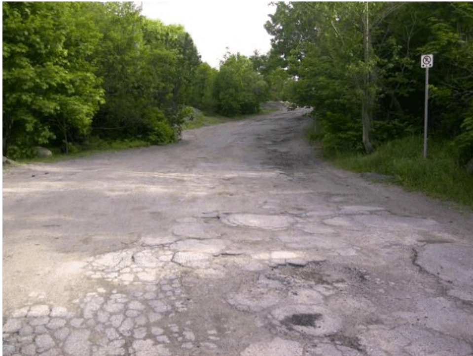
Photo 5 FROM FACER STREET LOOKING SOUTH ALONG DRIVEWAY ON/ADJACENT TO BELL PARK
