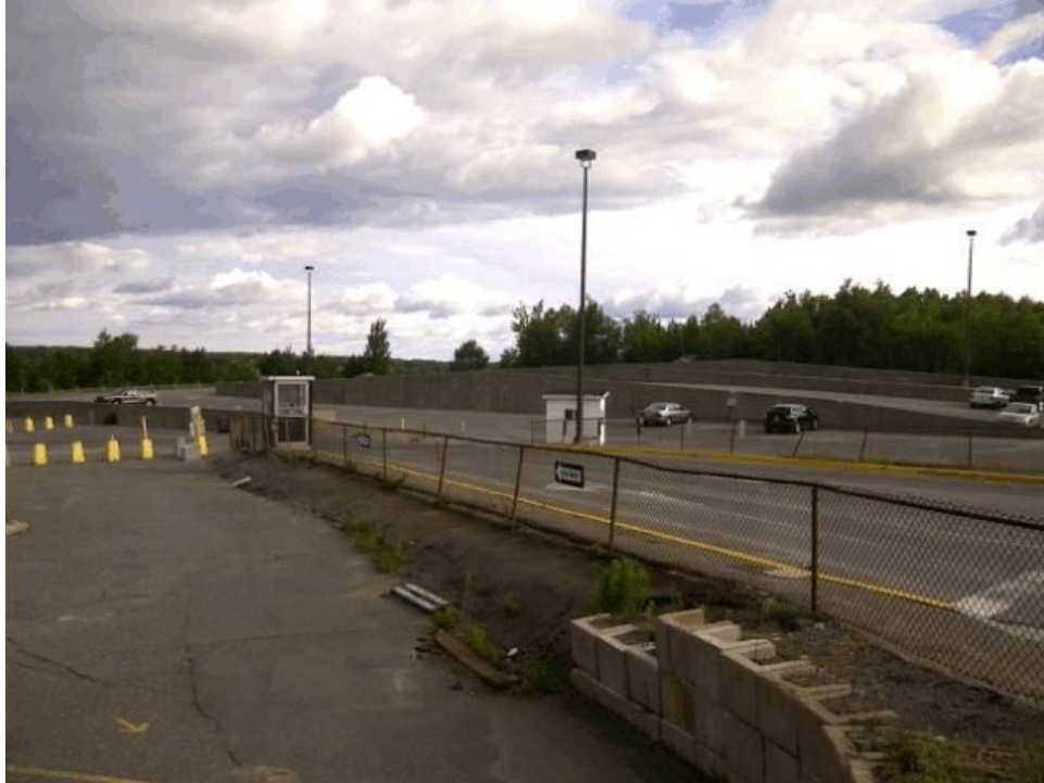
Photo 9 FROM PARIS STREET LOOKING TOWARDS THE CITY OWNED PARKING LOT LOCATED TO THE SOUTH OF THE SUBJECT LANDS
