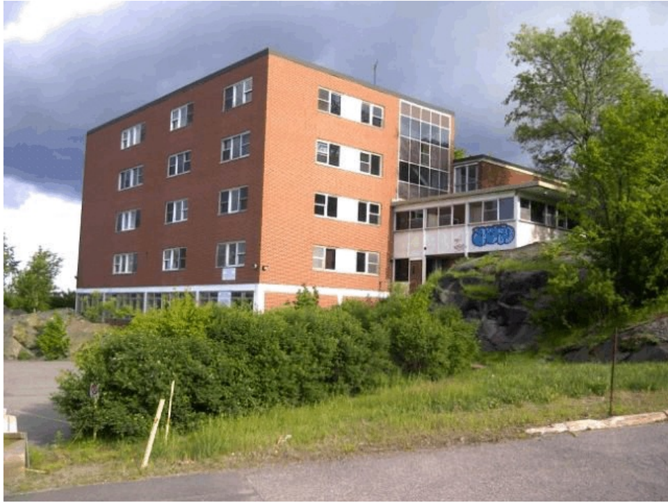
Photo 3 FORMER MASON RESIDENCE BUILDING (PROPOSED TO BE DEMOLISHED) LOCATED AT THE NORTH PART OF THE SITE
