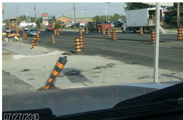
Inferior Asphalt Removed Next Day
