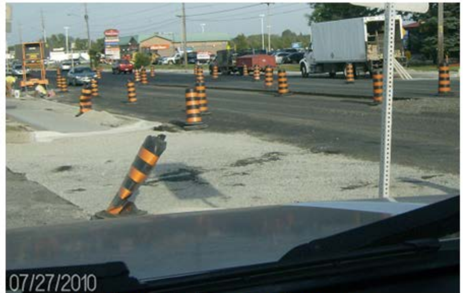
Inferior Asphalt Removed Next Day
