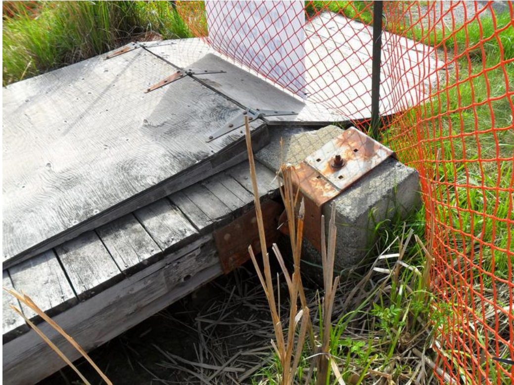
Photo 9 – Start of boardwalk and connection to abutment.
