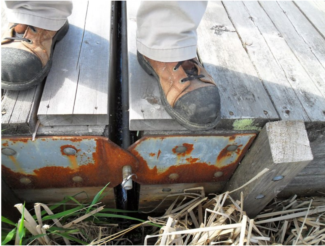
Photo 5 – Panel connection showing mild corrosion.
