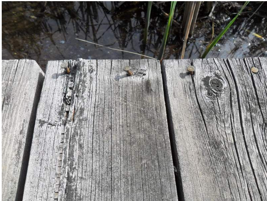
Photo 4 – Nail heads protruding
