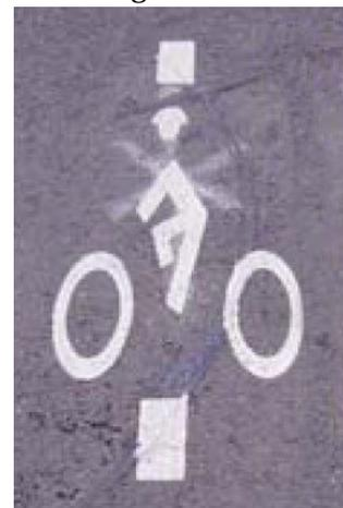
FIGURE 2—MARKING TO IDENTIFY TRAFFIC SIGNAL SENSOR IN PORTLAND, OR
