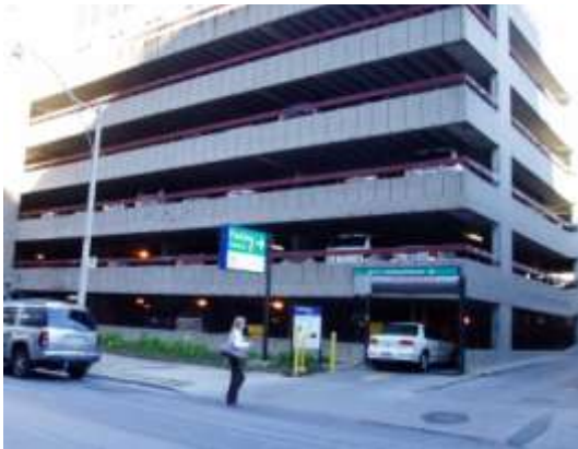
1. Parking garage with no urban design considerations (poor design)
