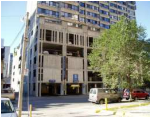
3. Parking garage with integrated residential development (good design)
