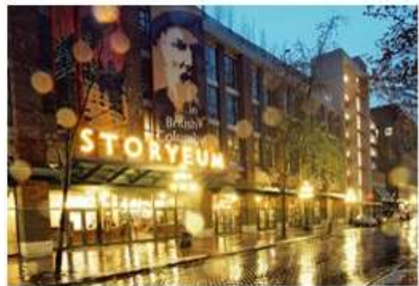
4. Parking garage with integrated retail (good design)
