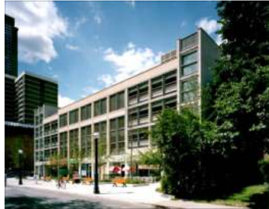
2. Parking garage with pedestrian amenities (good design)
