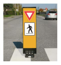
The bollard is set up in the middle of the street to increase the visibility of the crossover and to remind motorists to yield to pedestrians. Staff compared the compliance at all Type D locations before and after the installation of the bollards to see if they were effective. The table below shows the results for each location.
