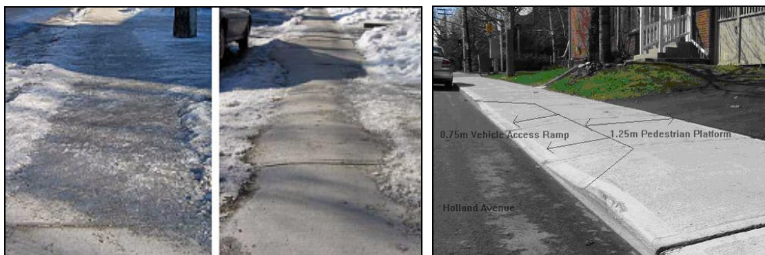
Figure 7. Flat-top sidewalk design currently utilised in Toronto, ON and Ottawa, ON.
