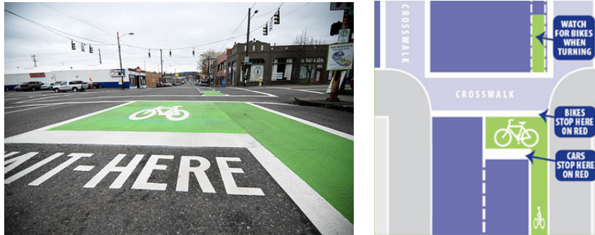
Figure 17. “Bike-Box” infrastructure allow bicycles to wait at traffic lights ahead of cars, to improve visibility.
