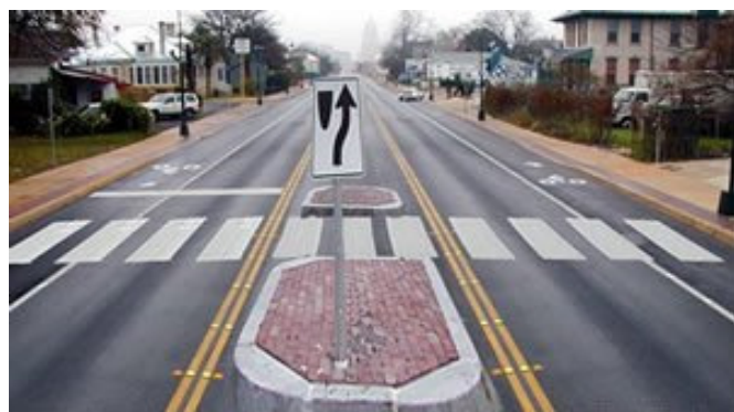
Figure 23. New road diet demonstrating the conversion of a formerly 4-lane thoroughfare to a complete street, with sidewalks, bicycle lanes and a pedestrian refuge island.
