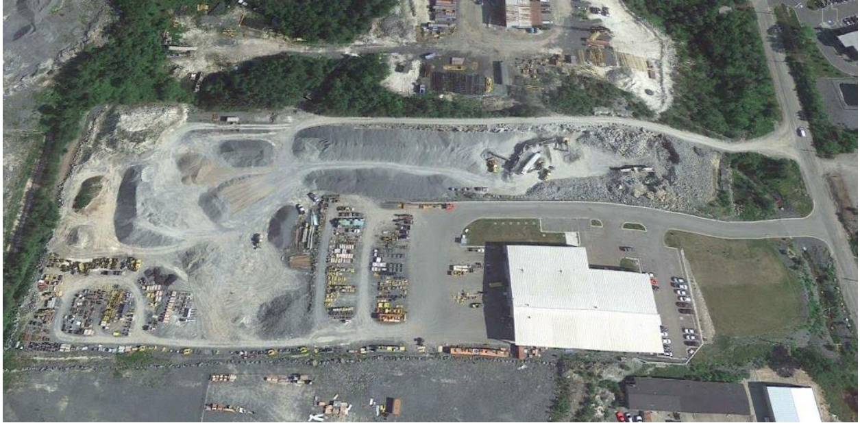
Photo 1: 234 & 240 Fielding Road, Lively Aerial photo dated July 2, 2019 illustrating extent of site alteration on PIN 73372-0232 and existing industrial facility on PIN 73372-0231 File 751-8/20-2 Source: Google Earth
