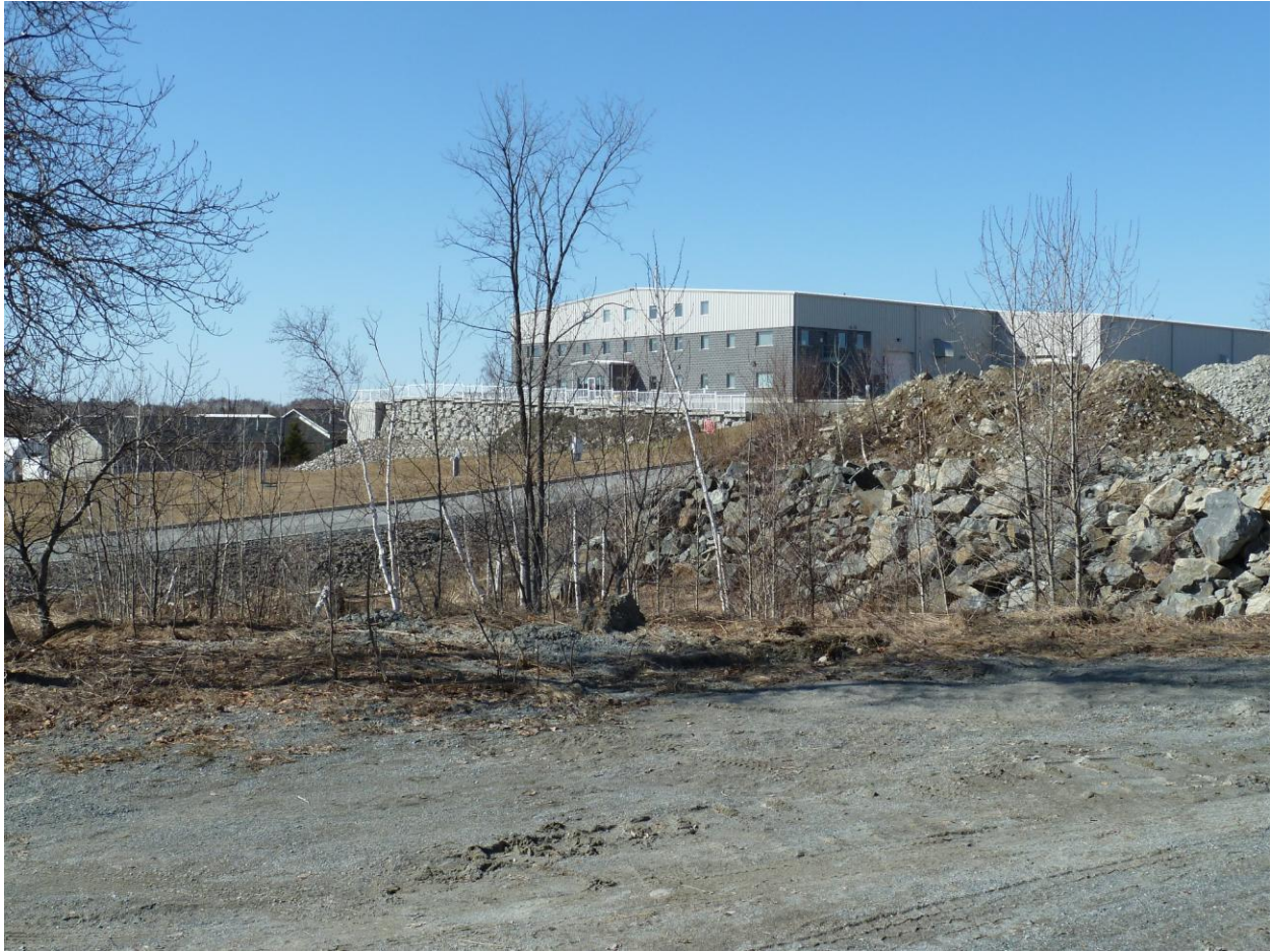
Photo 6: 240 Fielding Road, Lively Property benefitting from lot addition (Industrial Holdings) File 751-8/20-2 Photography April 11, 2020
