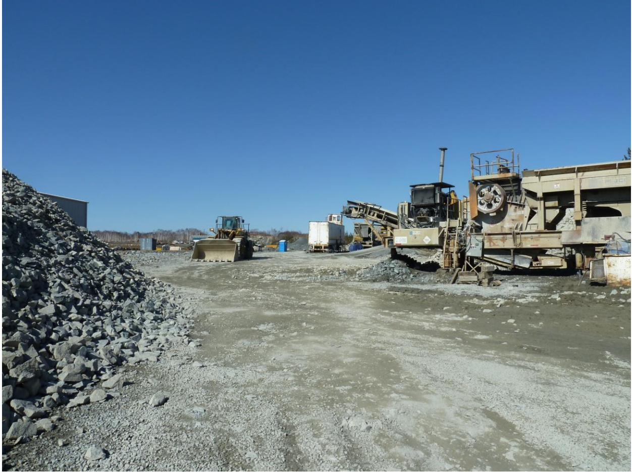
Photo 3: 234 Fielding Road, Lively Site alteration and heavy equipment on PIN 73372-0232 (Rintala Construction) File 751-8/20-2 Photography April 11, 2020
