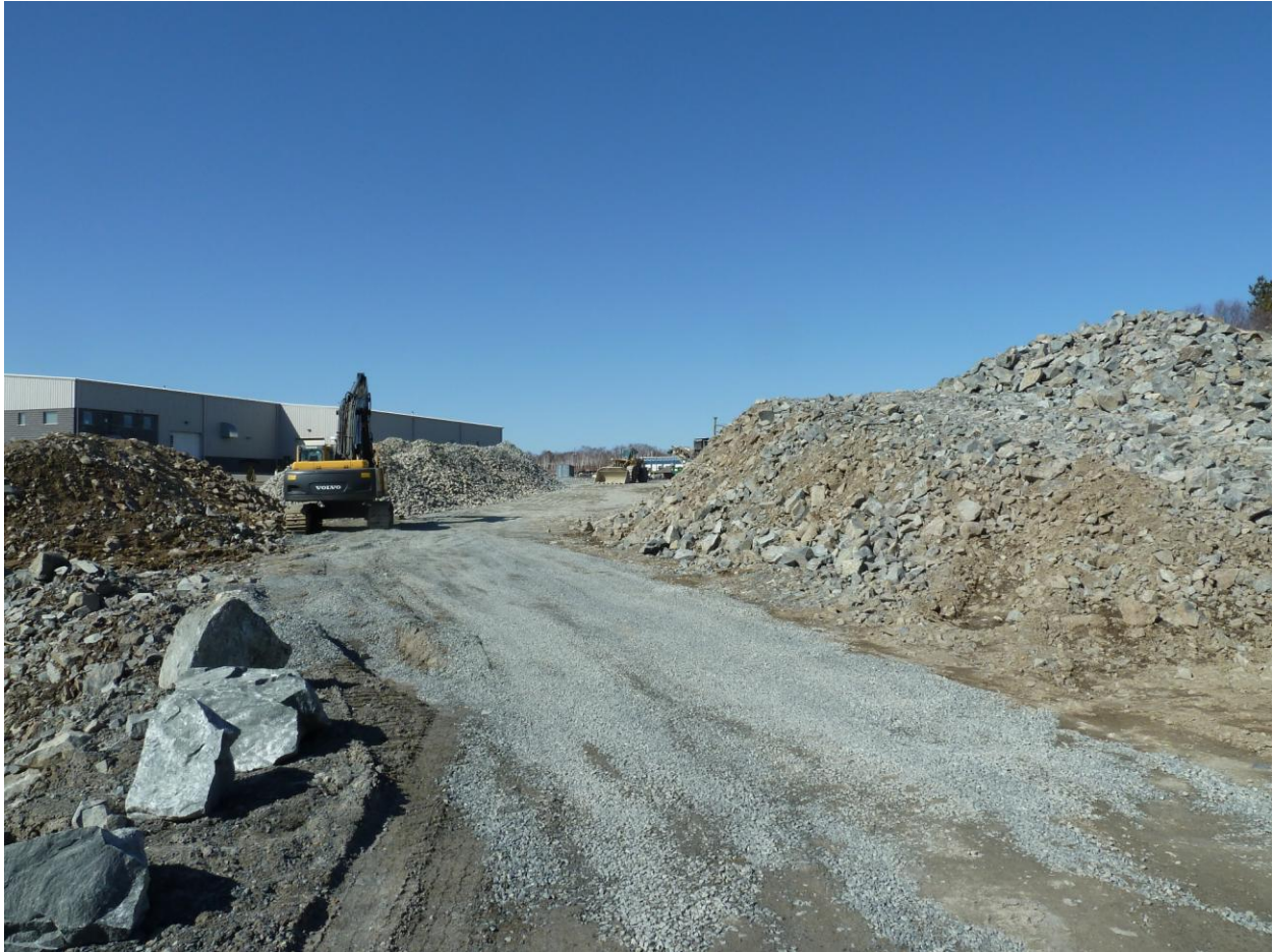
Photo 2: 234 Fielding Road, Lively Existing site conditions on PIN 73372-0232 (Rintala Construction) File 751-8/20-2 Photography April 11, 2020
