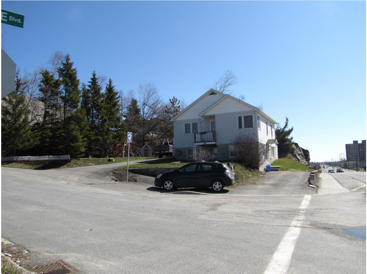
Photo #7. Existing residential structure at 1154 Northway to the east of the subject lands, looking east. Photo taken May 1, 2020.
