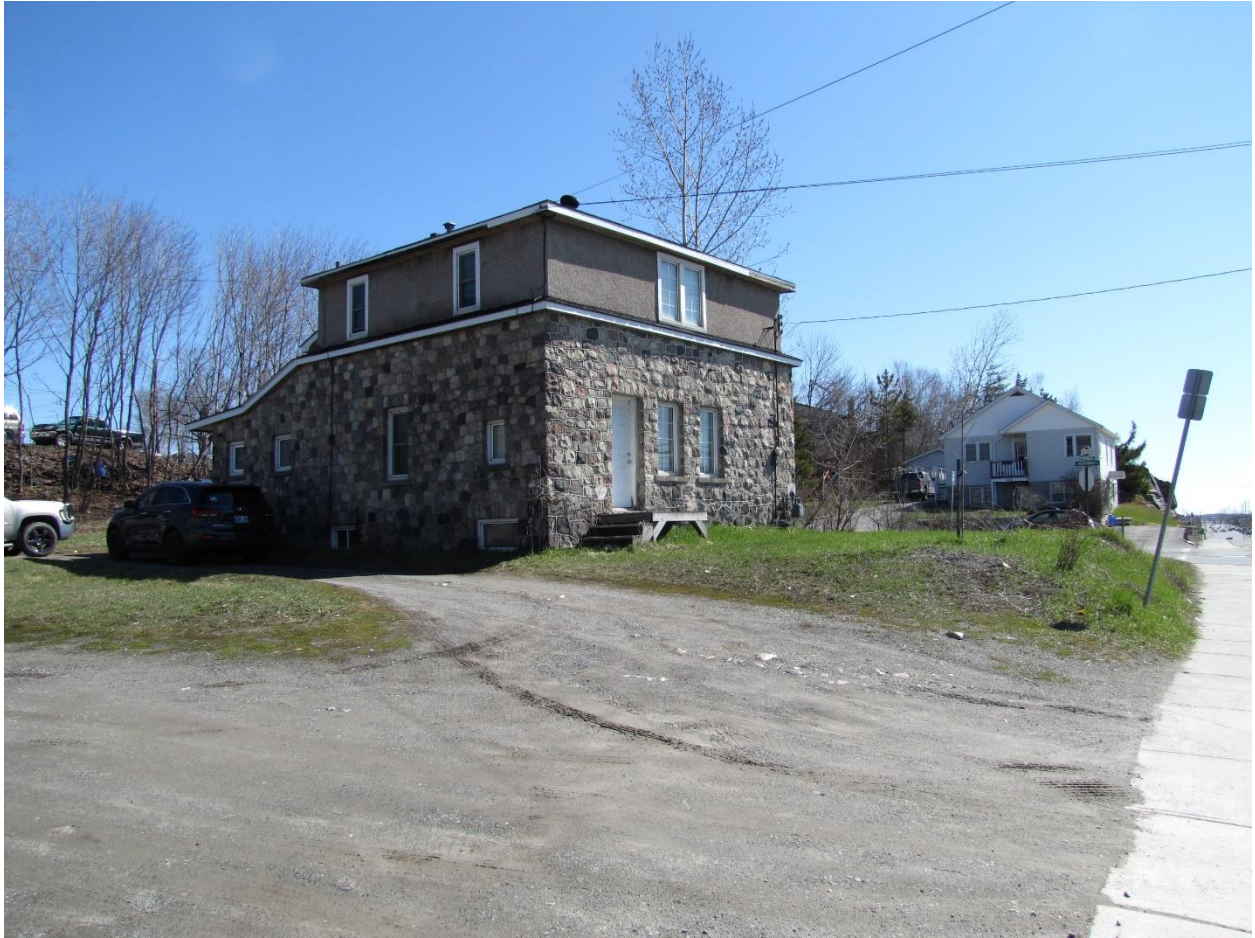
Photo #4. Corner of Northway and Lasalle, looking northeast. Photo taken May 1, 2020.
