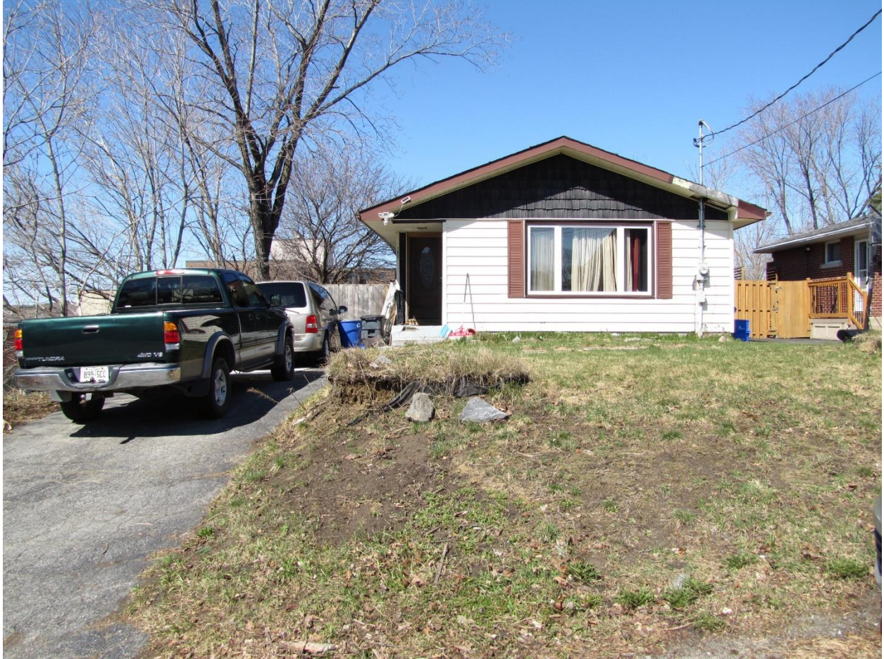
Photo #5. Existing residential structure at 1167 Northway, looking west. Photo taken May 1, 2020.
