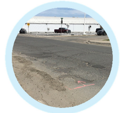
Example of Pavement Distress and Appropriate Candidate for Large Asphalt Patch
