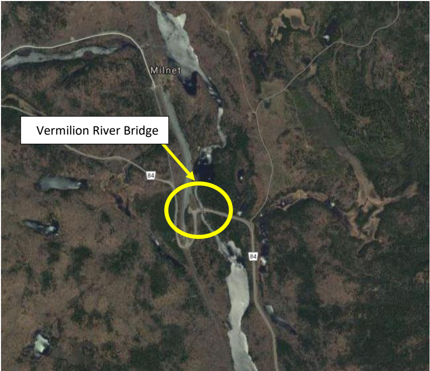
Image 2 – Vermilion River Bridge Location
