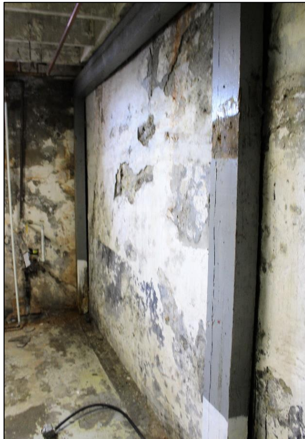
Figure 35: Deflection of north wall (Source: ML 2020).
