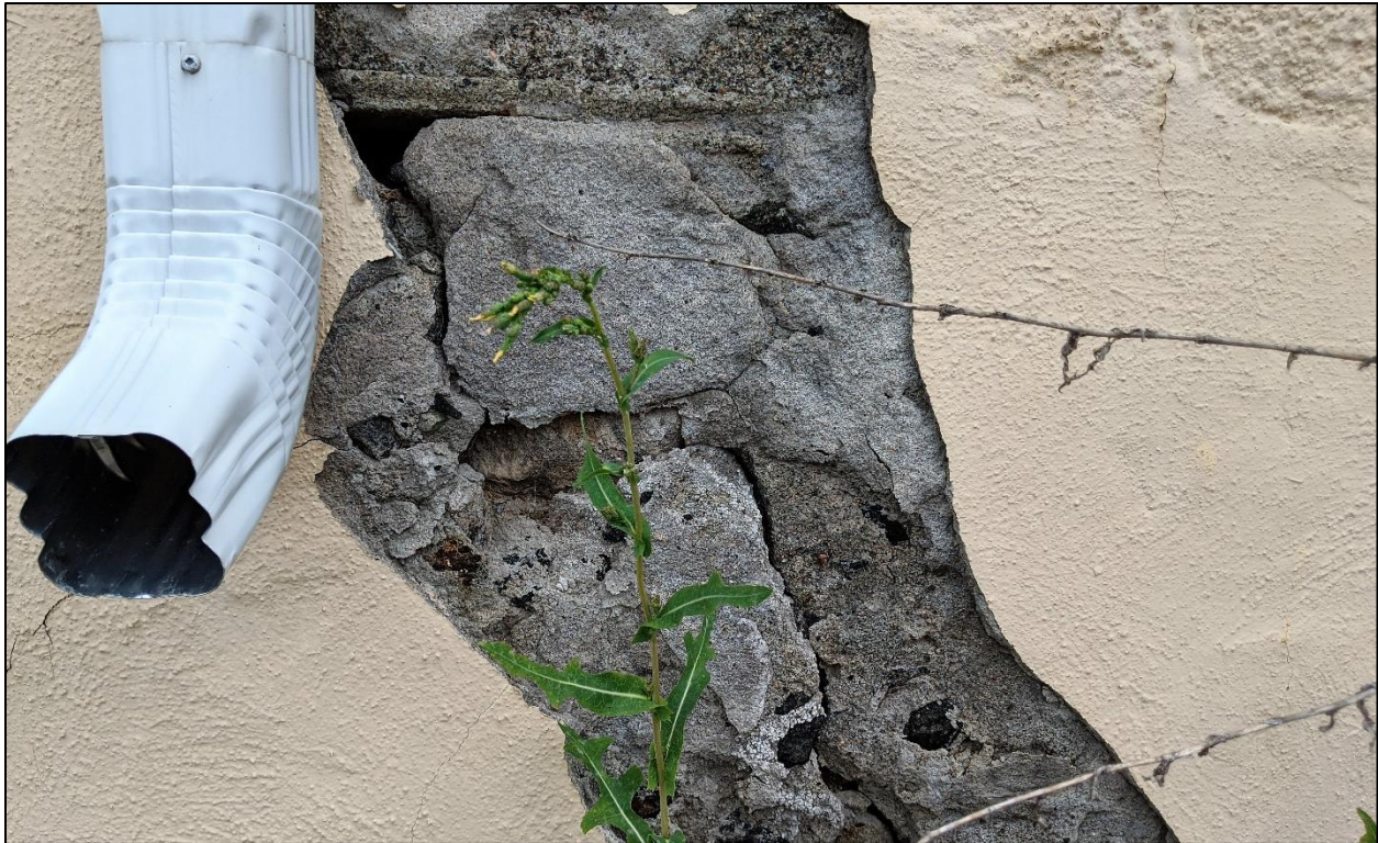
Figure 24: Exposed concrete rubble foundations covered in parging on the northwest corner (Source: ML, 2020).
