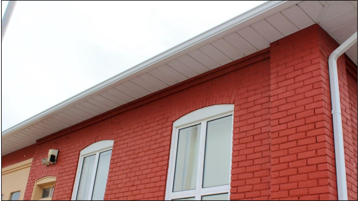
Figure 29: Detail of the northern elevation windows with brick voussoirs (Source: ML, 2020).
