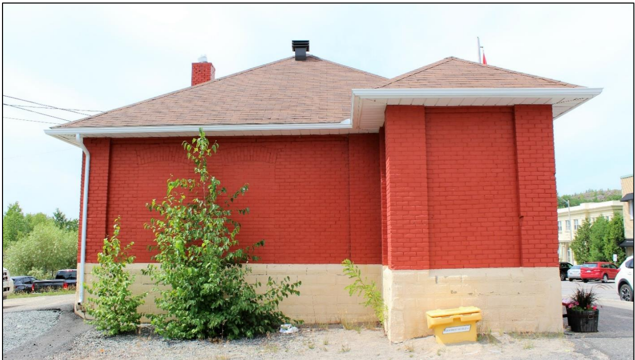
Figure 28: East elevation showing the two sealed windows and the base of the decommissioned hose tower (Source: ML, 2020).
