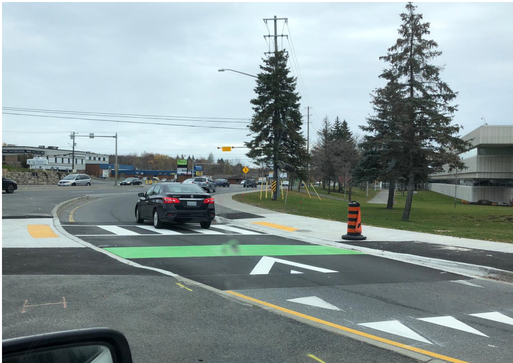
Figure 3. New raised pedestrian and cyclists crossing and pavement markings in the right-turn channel from Notre Dame Avenue to LaSalle Boulevard
