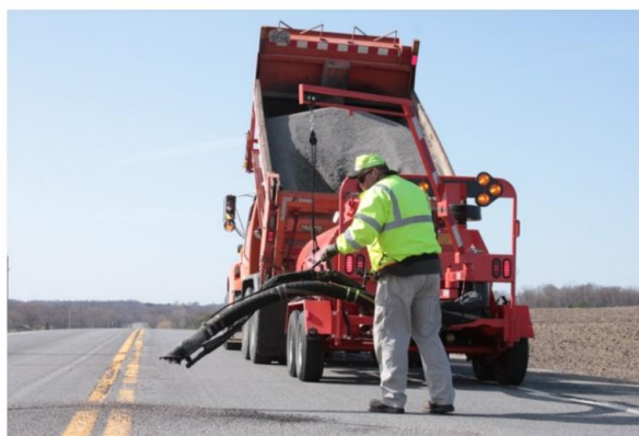
Figure 3 – Trailer-mounted Spray Patcher (Transportation Association of Canada, Best Practices in Pothole Repair - 2019)
