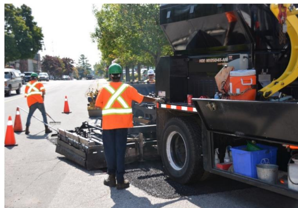
Figure 5 – Trailer-mounted infrared unit (Transportation Association of Canada, Best Practices in Pothole Repair - 2019)
