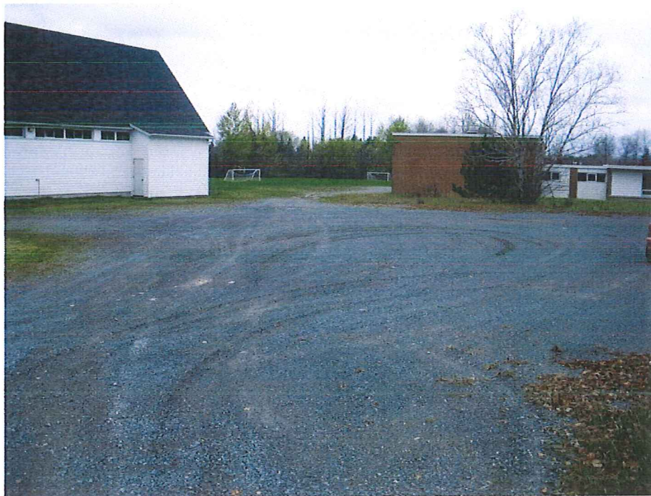
PHOTO 2 EXISTING PARKING AREA TO THE NORTH OF THE EXISTING BUILDING LOOKING WEST FROM MARY AVENUE
