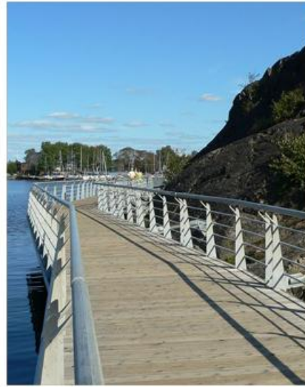
BELL PARK BOARDWALK
