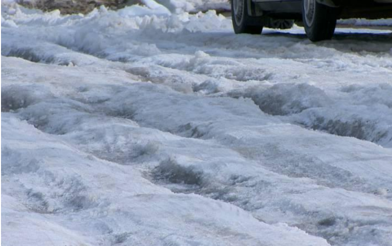
Picture 3 – Severe Ice Ruts
