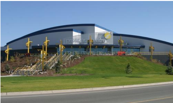
Figure 19 Prospera Centre, Chilliwack BC (2004)
