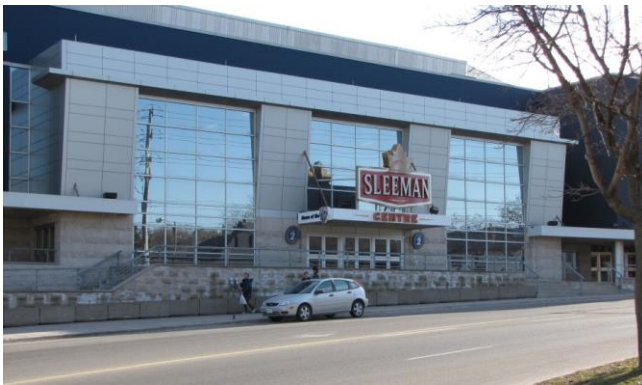
Figure 22 Sleeman Centre, Guelph ON (2000)
