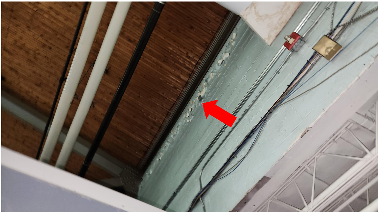
Photo 28: Peeling paint on masonry wall (c.1951).
