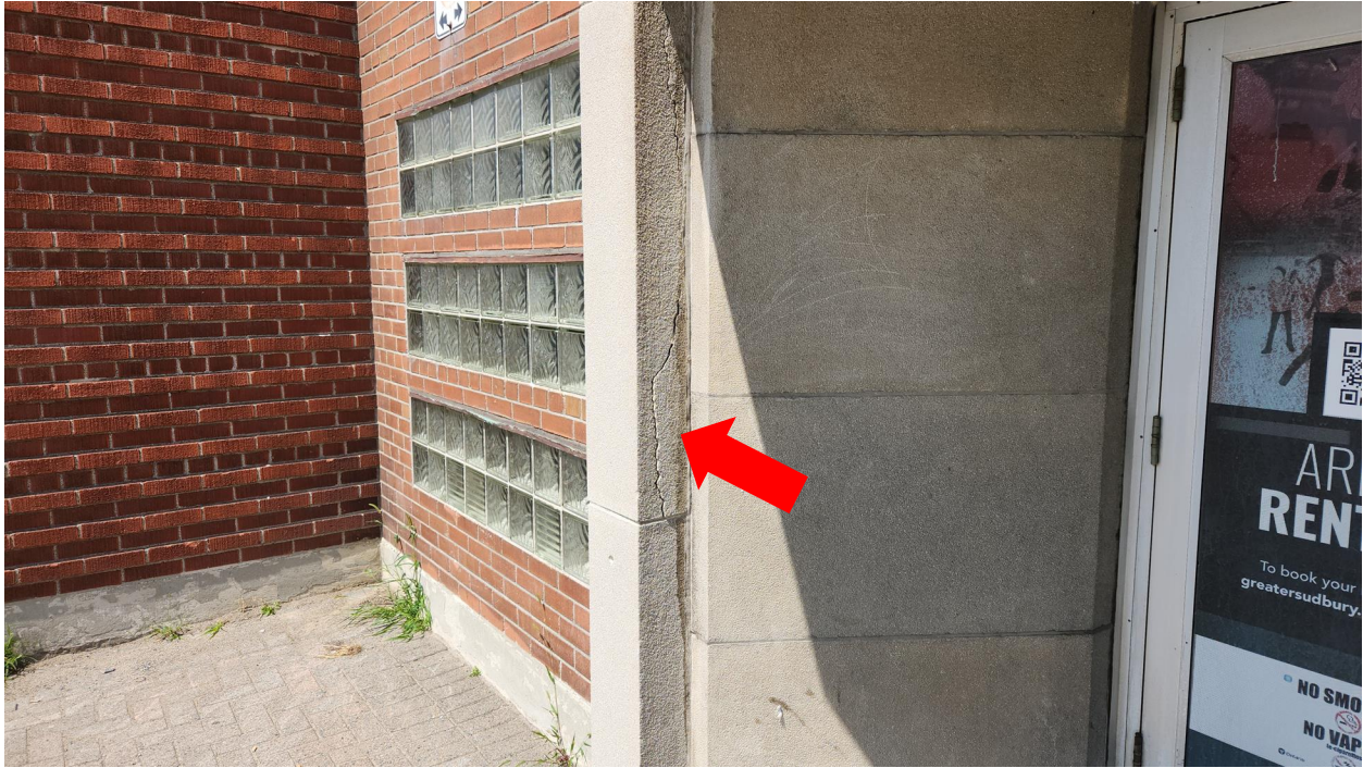
Photo 35: Cracked precast concrete at Main Entrance (c.1951).
