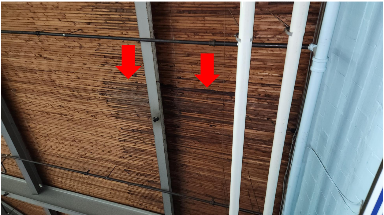
Photo 4: Water stains at underside of NLT deck (High Roof c.1951).
