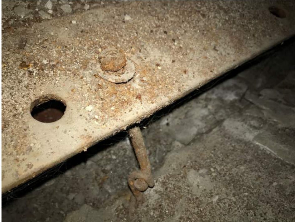
Figure 9: Typical soffit anchor j-bolt. Surface corrosion and nut not fully threaded.
