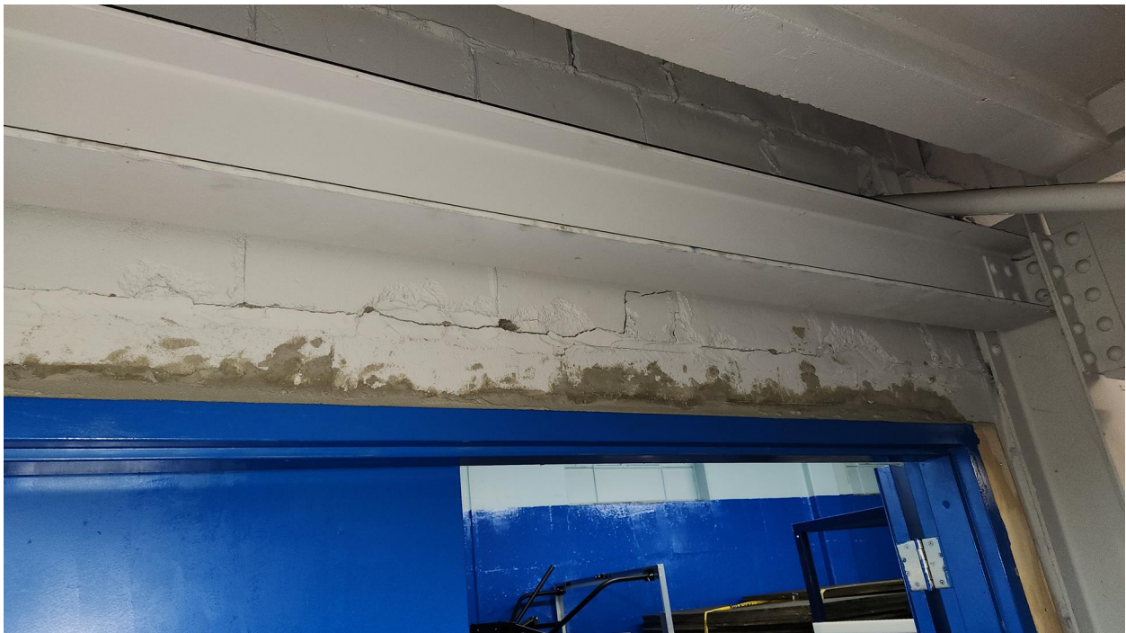
Photo 30: Missing lintel over Storage Room door (c.1951).
