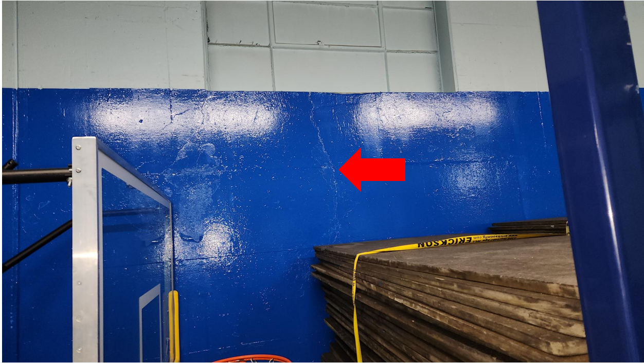
Photo 17: Typical crack in concrete foundation wall (c.1951).
