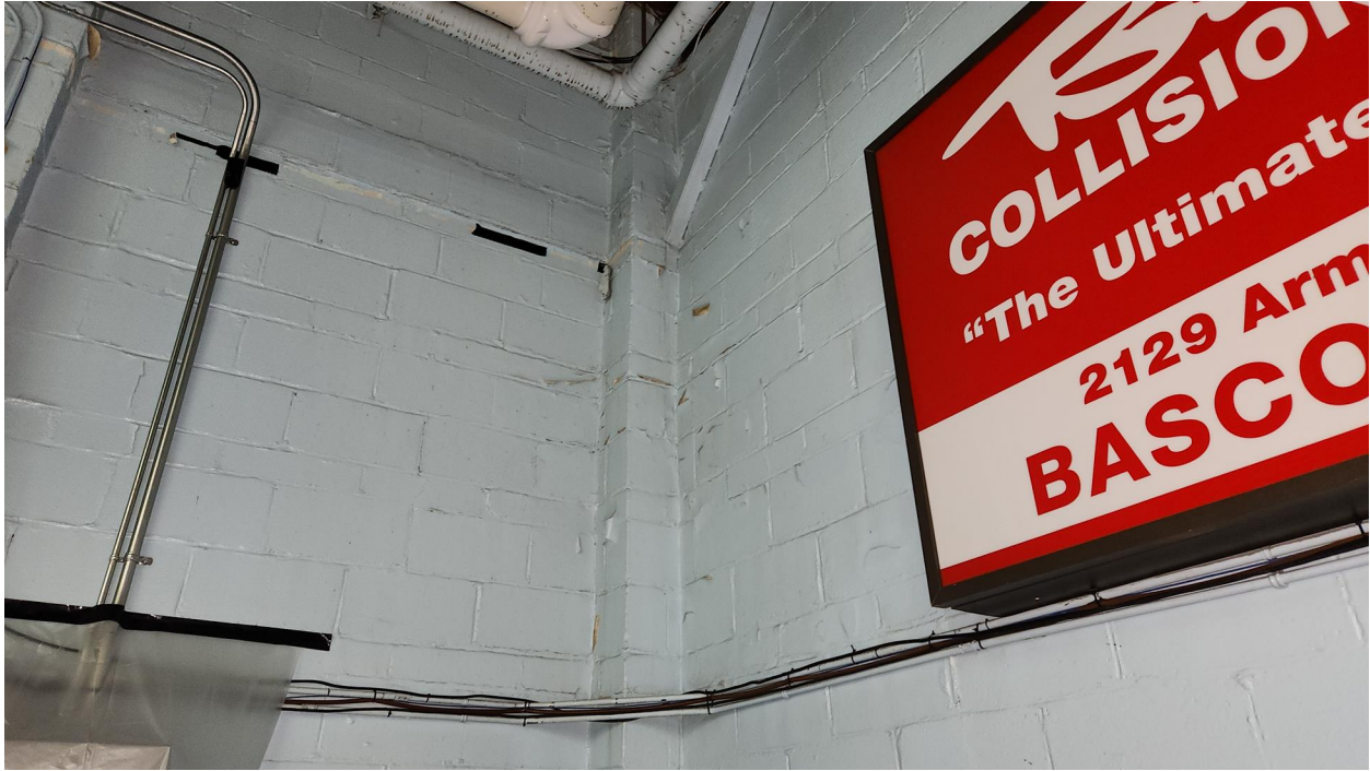
Photo 29: Peeling paint on masonry wall (c.1951).
