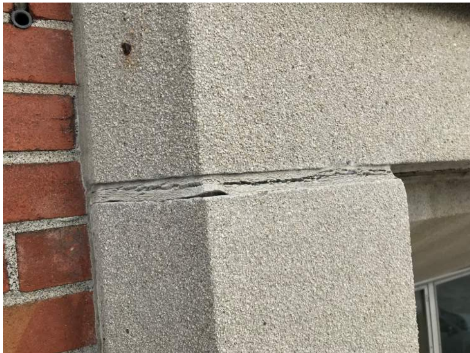
Figure 10: Typical sealant joint deterioration.
