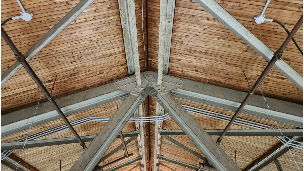
Photo 3: Typical High Roof structure exhibiting light surface corrosion (c.1951).
