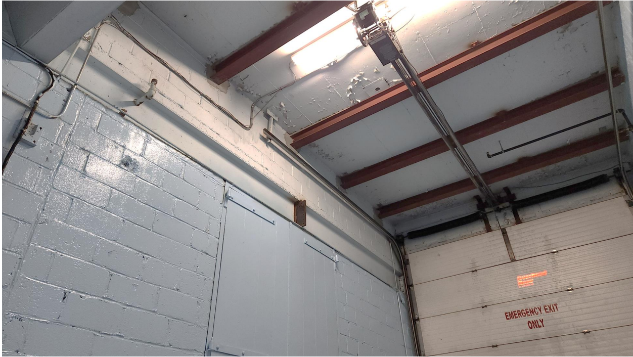
Photo 49: Steel beams below concrete slab believed to be installed as part of the c.2006 addition.
