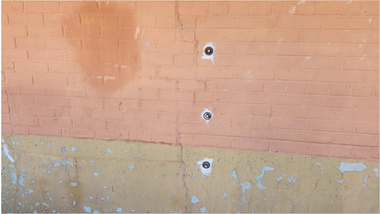
Photo 23: Crack in concrete foundation and masonry walls (c.1951).
