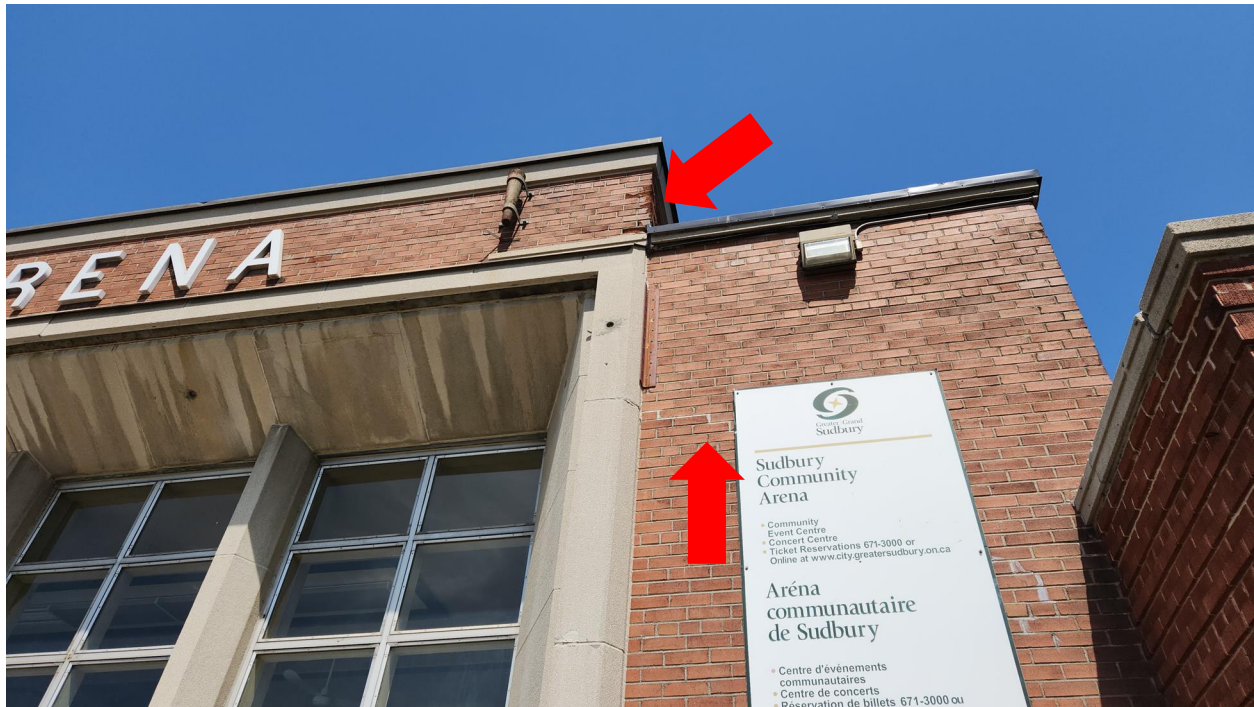
Photo 31: Damaged and cracked brick masonry (c.1951).
