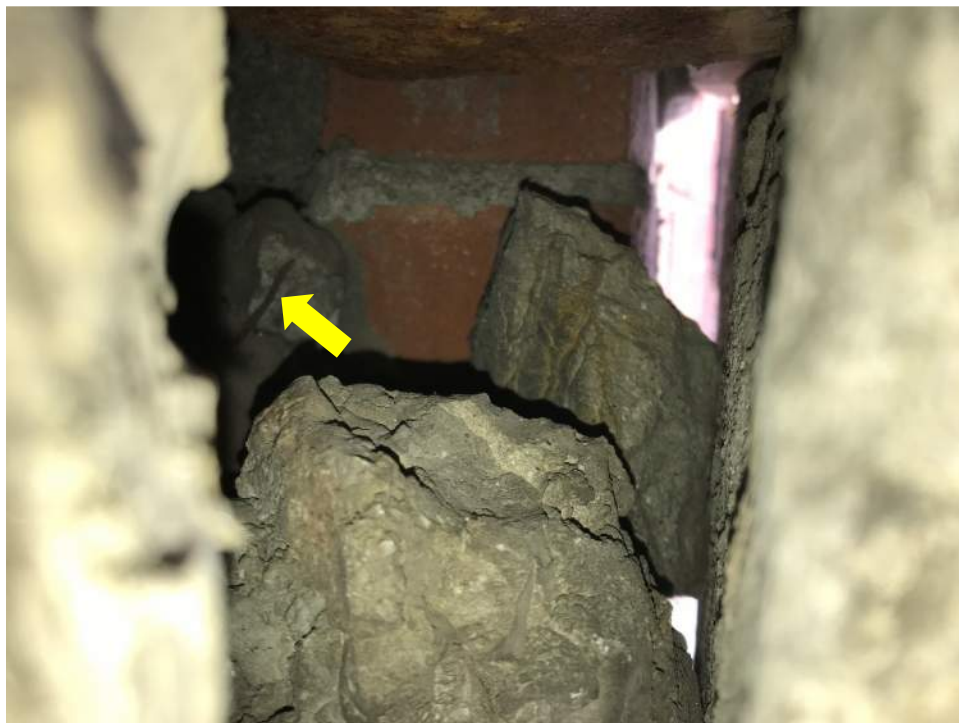
Figure 4: Typical snapped wire tie.
