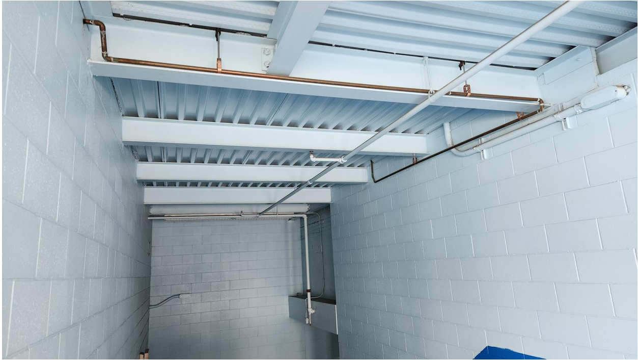
Photo 39: Typical floor framing (c.2000).
