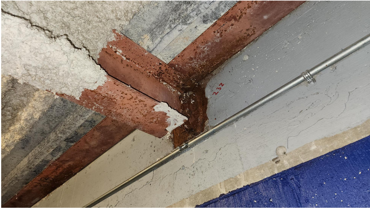
Photo 41: Corrosion of beam-to-column header connection at the southeast stair addition (c.2000).
