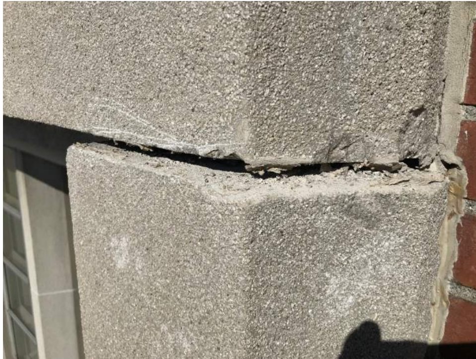
Figure 3: Typical displacement of topmost panel on outer column.
