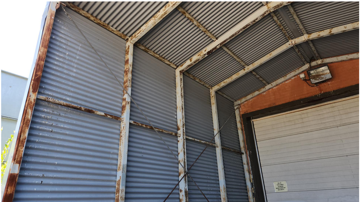
Photo 38: Condition of steel canopy.
