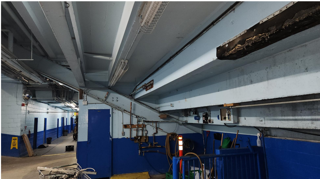
Photo 8: Typical Grandstand seating framing (c.1951).
