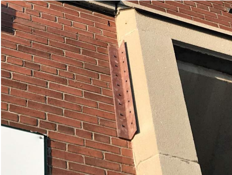
Figure 5: Immediate temporary panel support.
