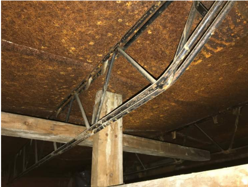
Figure 3: Typical OWSJ framing spanning between steel beams.
