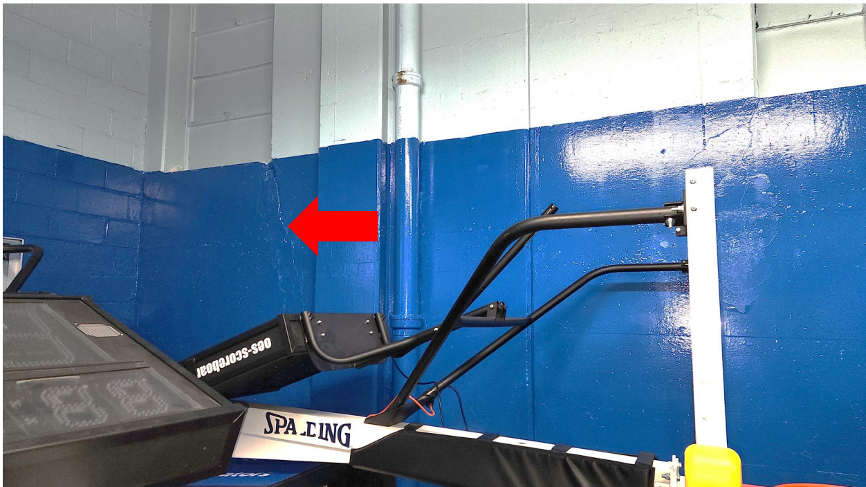
Photo 18: Typical crack in concrete foundation wall (c.1951).
