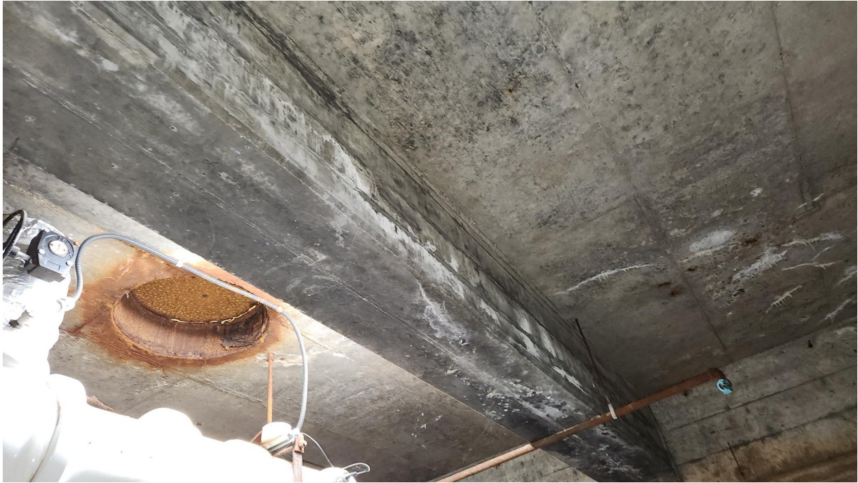
Photo 21: Evidence of water infiltration through roof slab in the old Coal Storage room (c.1951).
