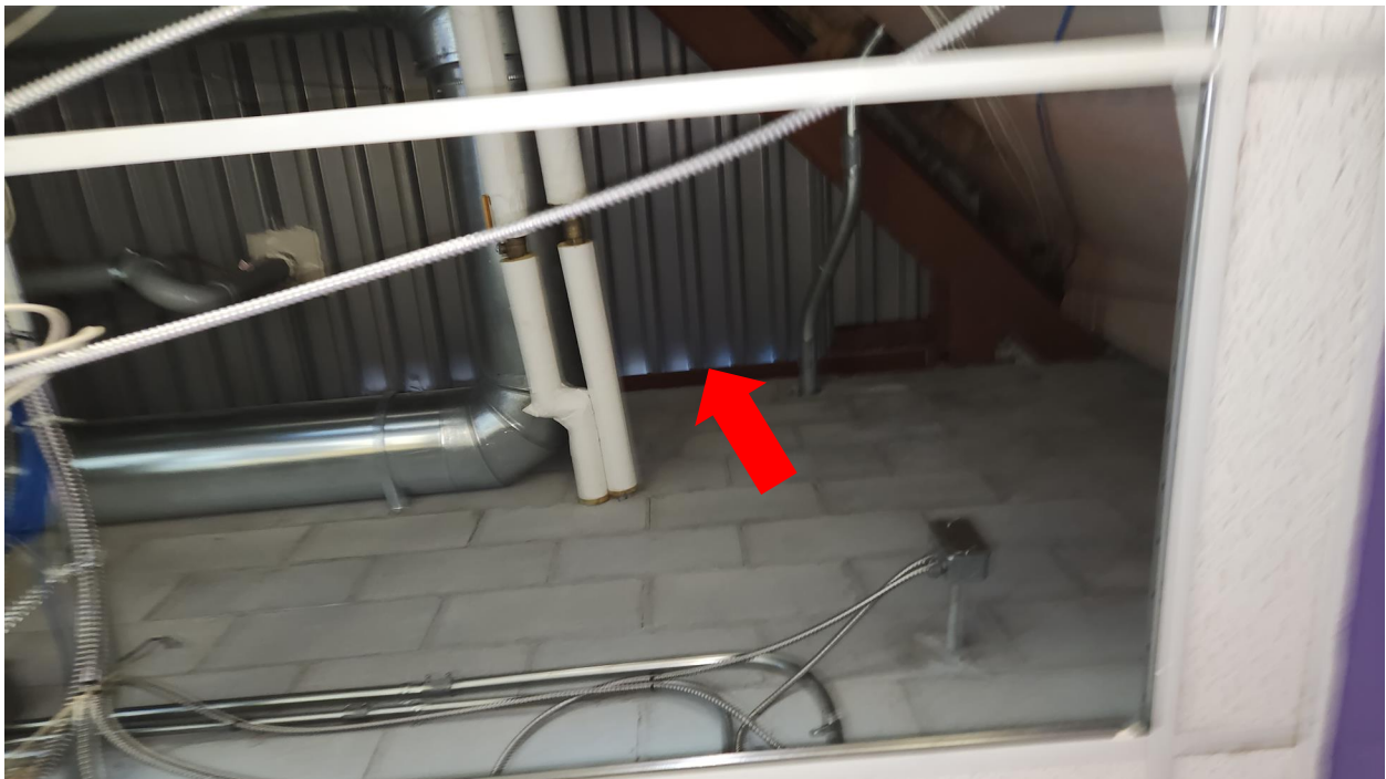
Photo 46: Gaps between the steel deck flutes and top of wall at the northwest stair addition (c.2000).
