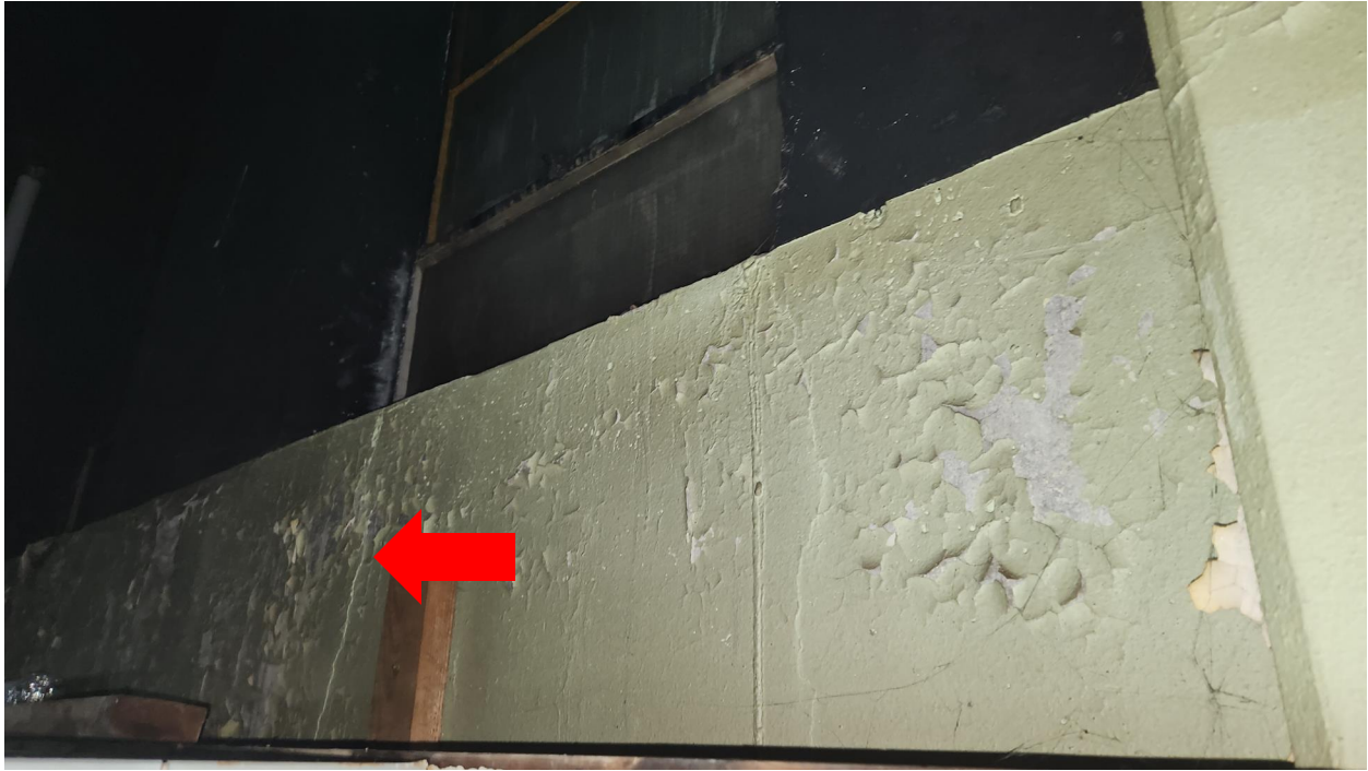
Photo 19: Typical crack in concrete foundation wall (c.1951).
