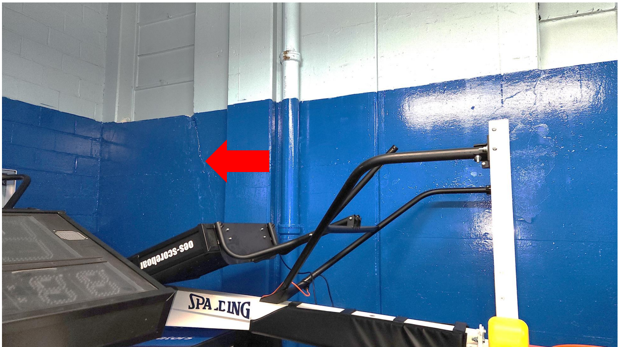
Photo 18: Typical crack in concrete foundation wall (c.1951).
