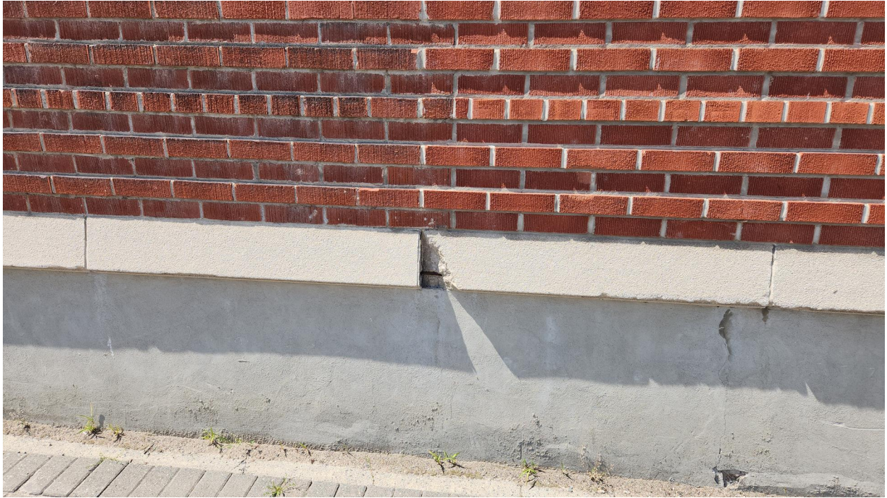
Photo 37: Damaged precast concrete sill (c.1951).
