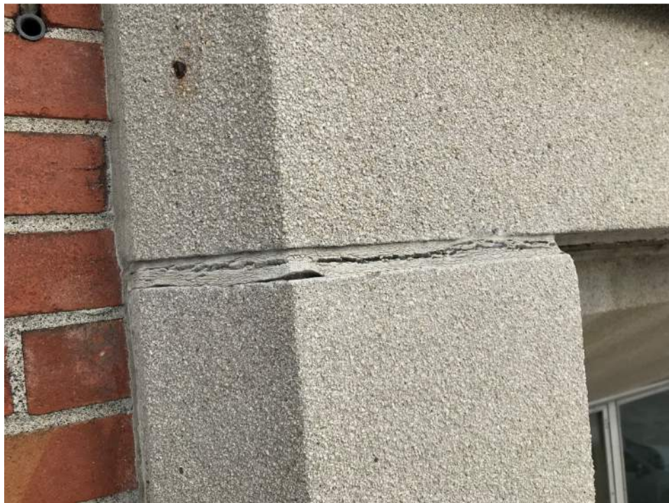
Figure 10: Typical sealant joint deterioration.
