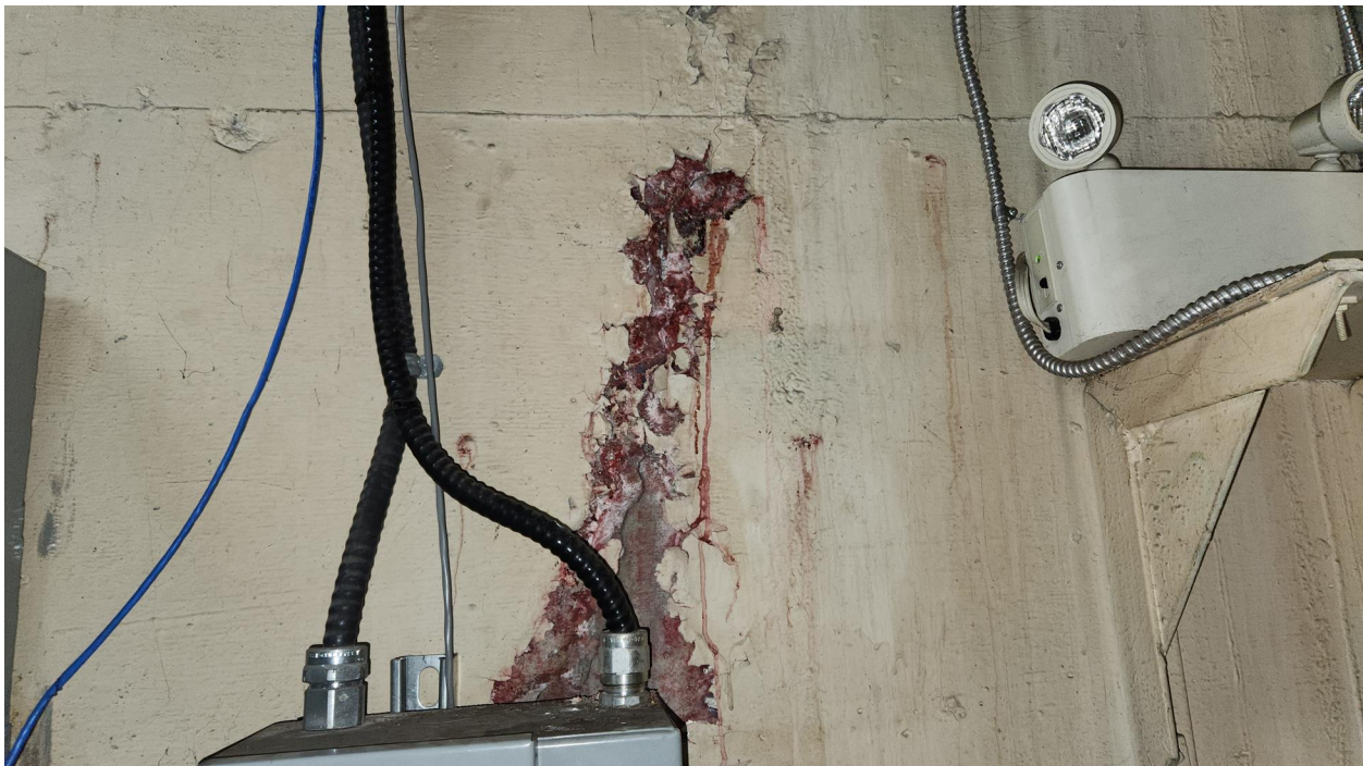
Photo 16: Evidence of leakage through concrete foundation wall in the Mechanical Room (c.1951).
