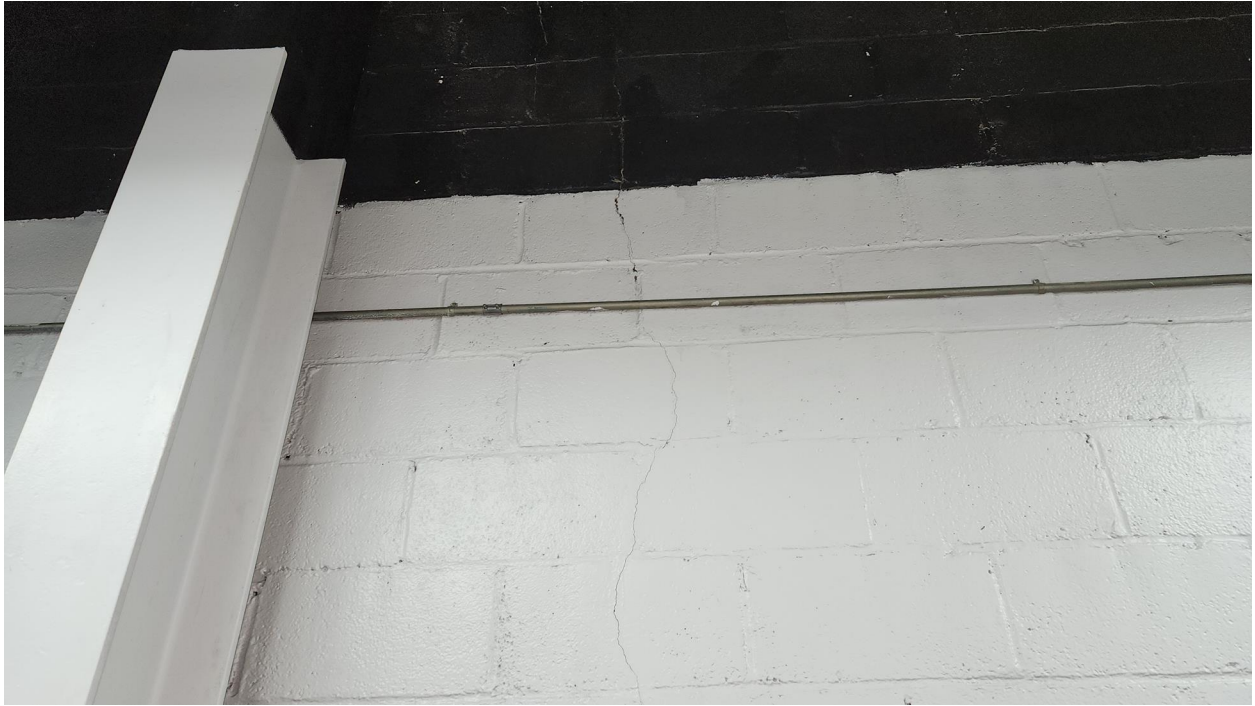
Photo 25: Crack in masonry wall (c.1951).
