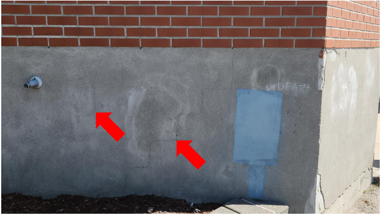
Photo 45: Step-cracking in masonry wall at the southwest stair addition (c.2000).
