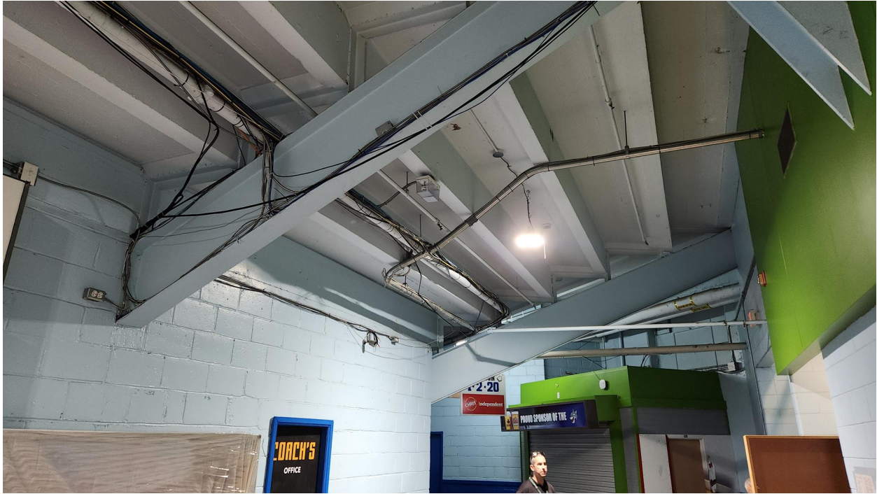
Photo 9: Typical Grandstand seating framing (c.1951).
