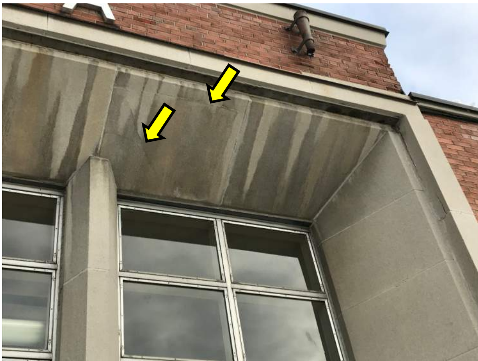
Figure 6: Soffit panel cracks and staining.
