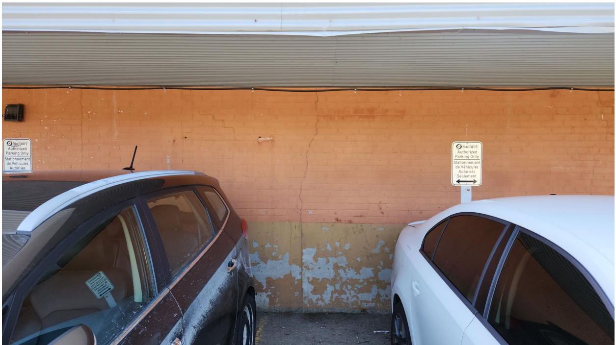
Photo 24: Cracks in concrete foundation and masonry walls (c.1951).
