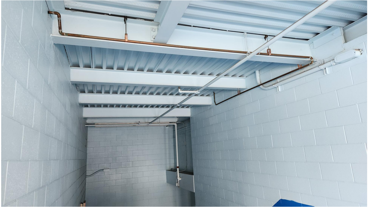
Photo 39: Typical floor framing (c.2000).
