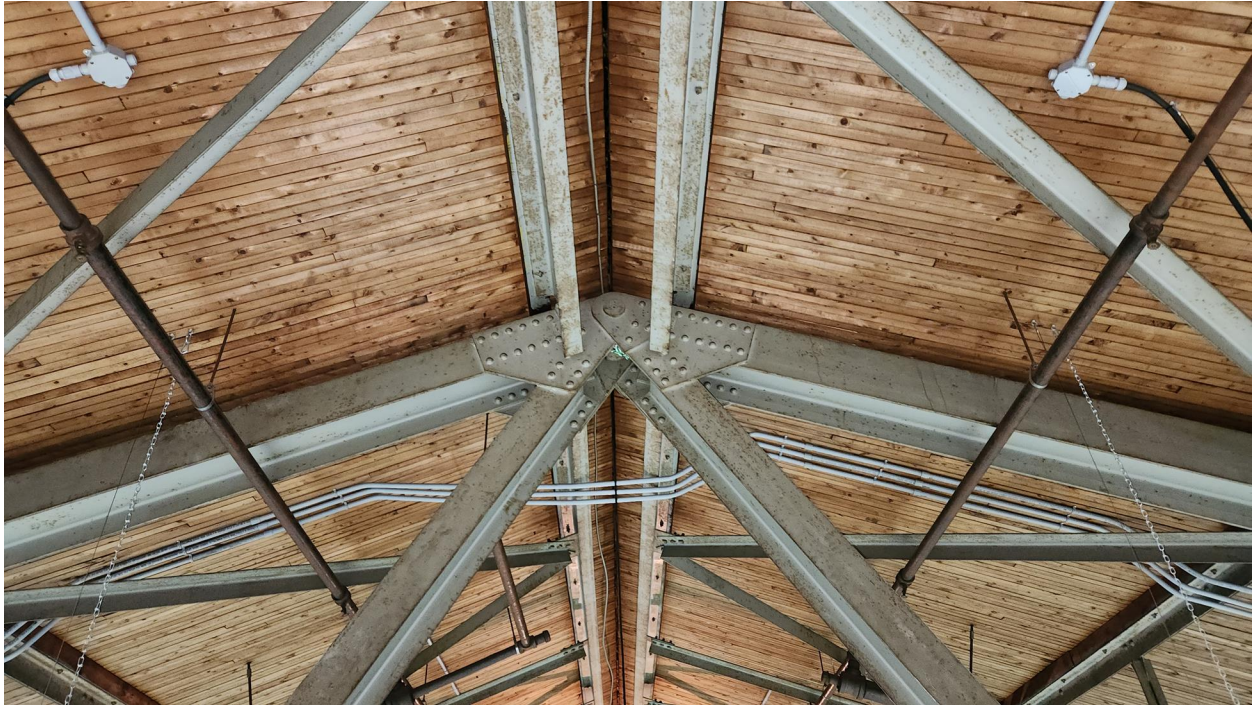
Photo 3: Typical High Roof structure exhibiting light surface corrosion (c.1951).
