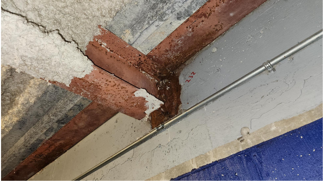
Photo 41: Corrosion of beam-to-column header connection at the southeast stair addition (c.2000).
