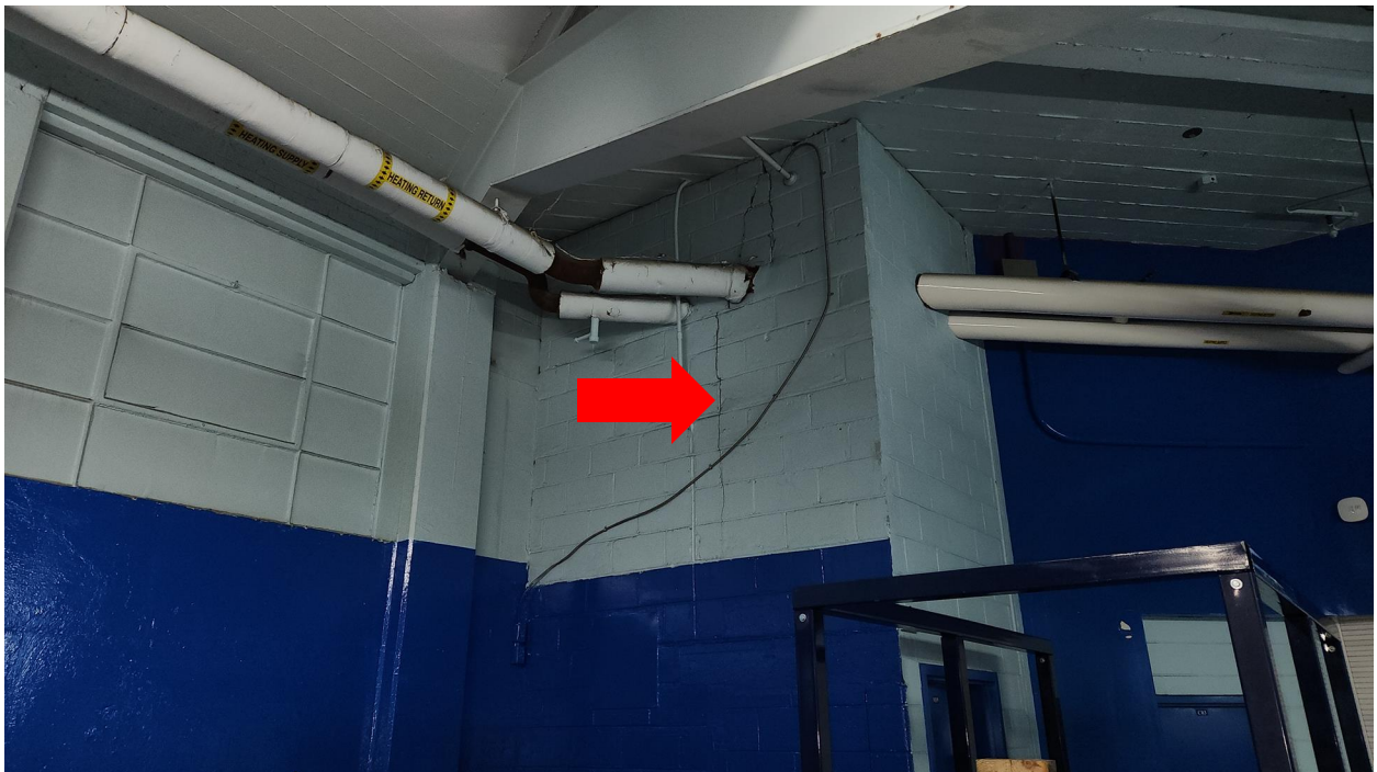
Photo 26: Crack in masonry wall (c.1951).
