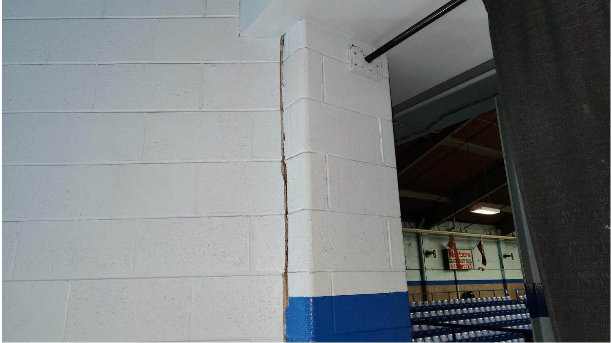
Photo 43: Masonry wall cracks at the southwest stair addition (c.2000).
