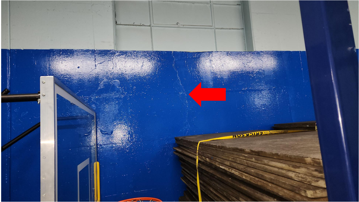
Photo 17: Typical crack in concrete foundation wall (c.1951).
