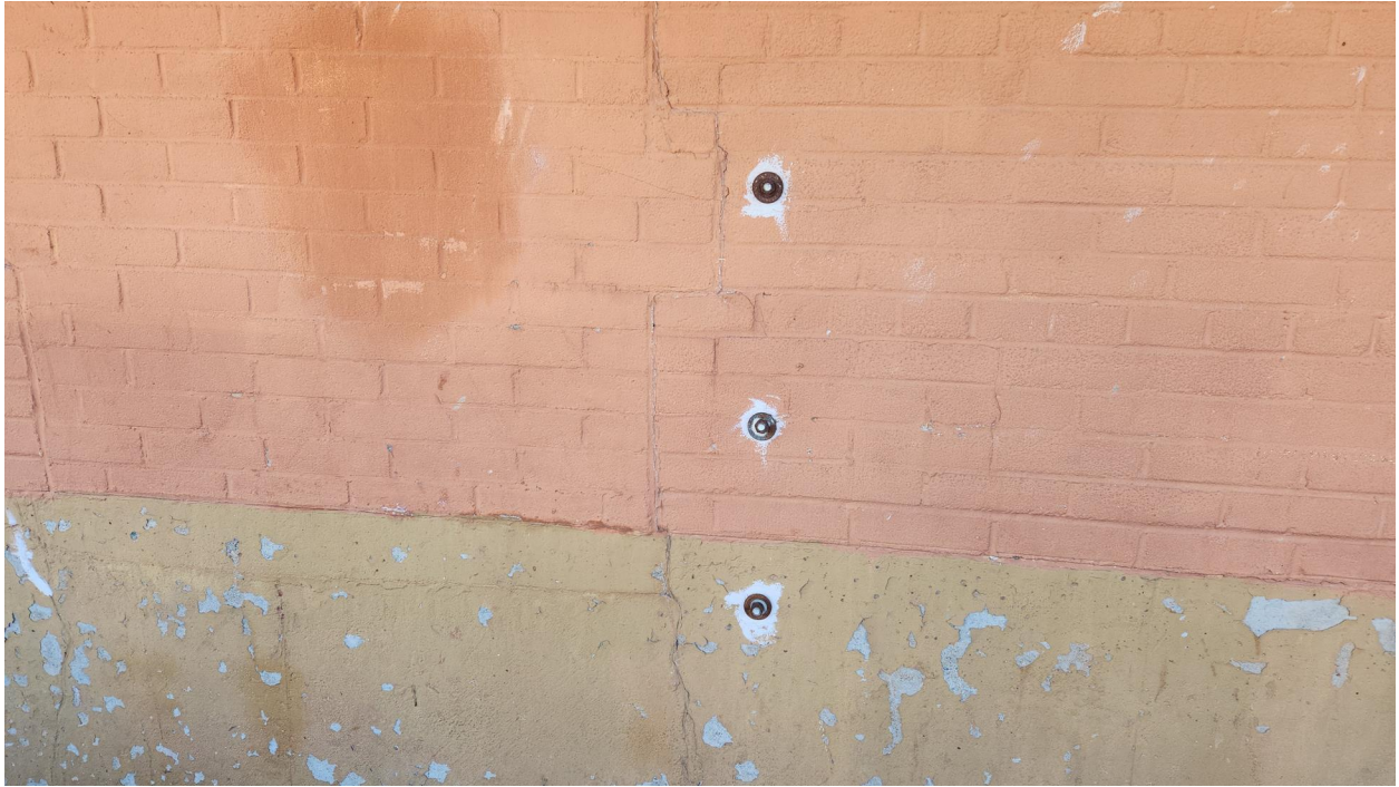
Photo 23: Crack in concrete foundation and masonry walls (c.1951).
