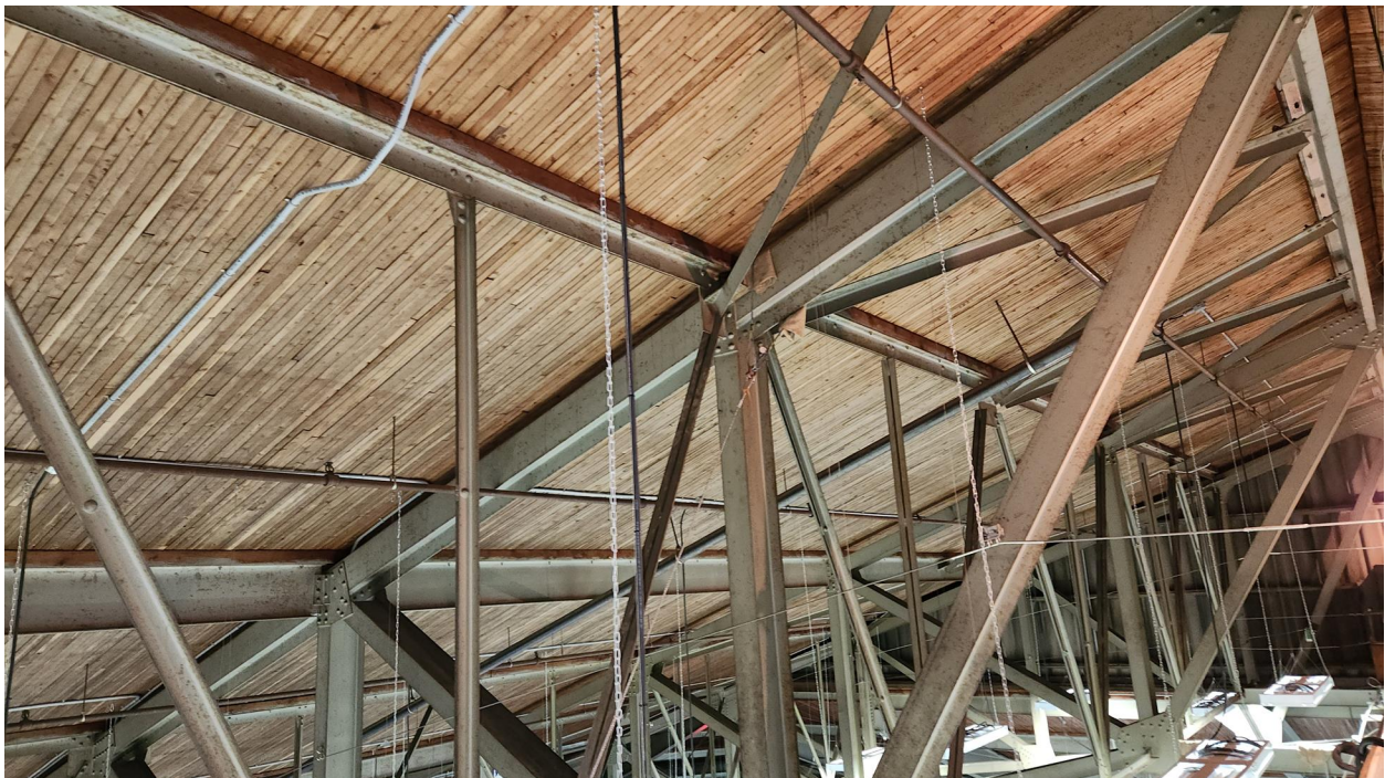
Photo 6: Typical High Roof structure exhibiting light surface corrosion (c.1951).
