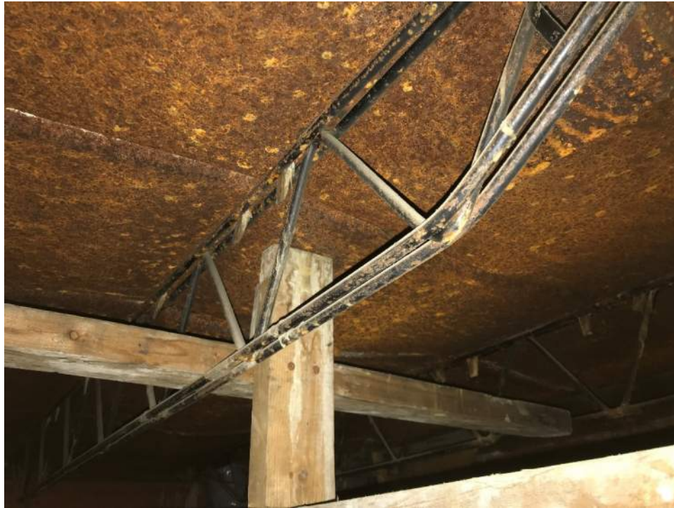
Figure 3: Typical OWSJ framing spanning between steel beams.
