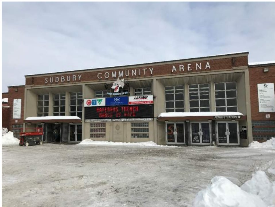
Figure 1: General view of main entrance precast concrete panels.
