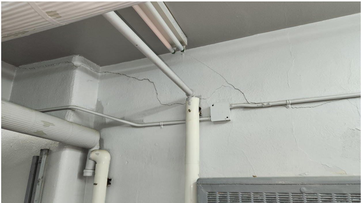
Photo 20: Cracked and spalling parging on the foundation walls at the south side of the building (c.1951).
