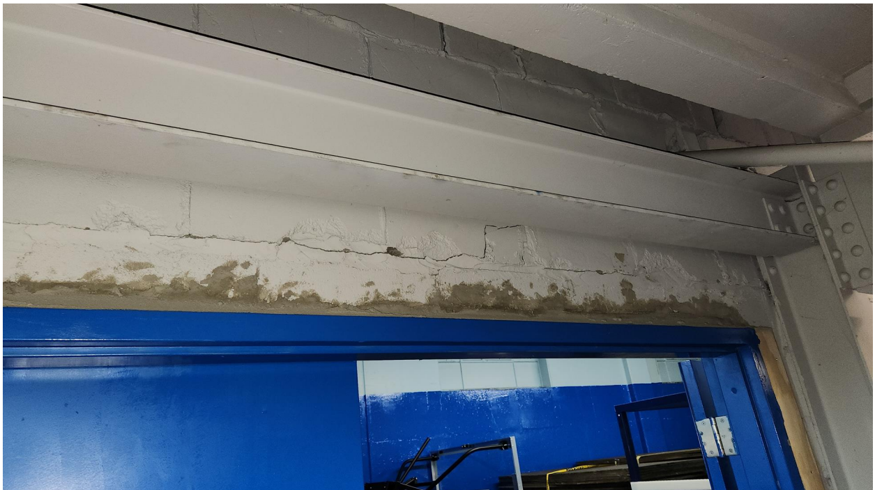
Photo 30: Missing lintel over Storage Room door (c.1951).
