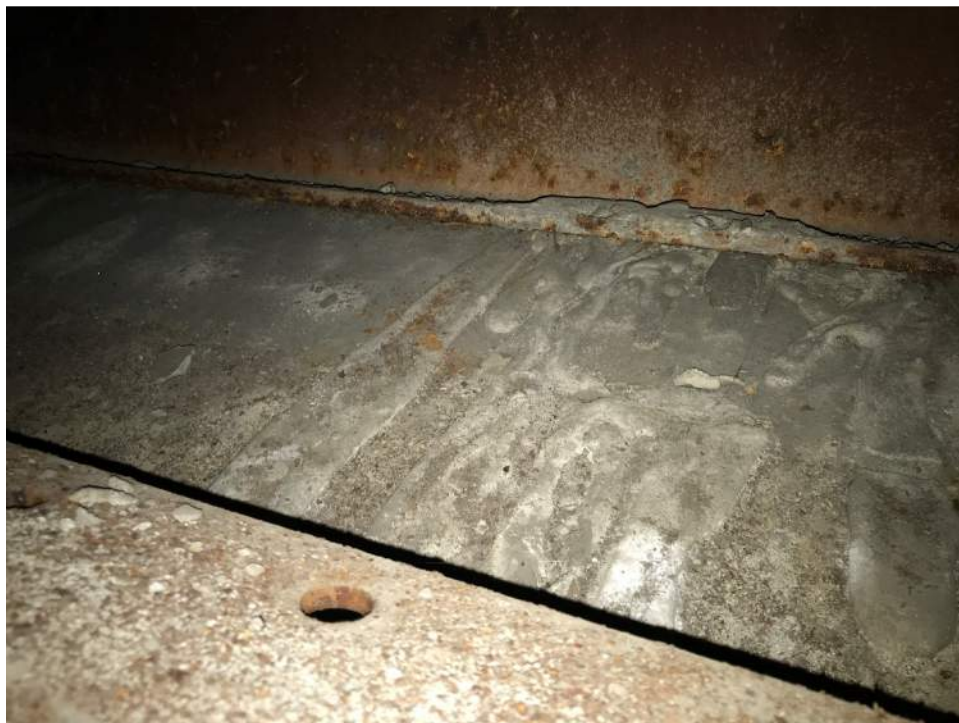
Figure 8: Surface corrosion and missing anchors at all pre-drilled holes.
