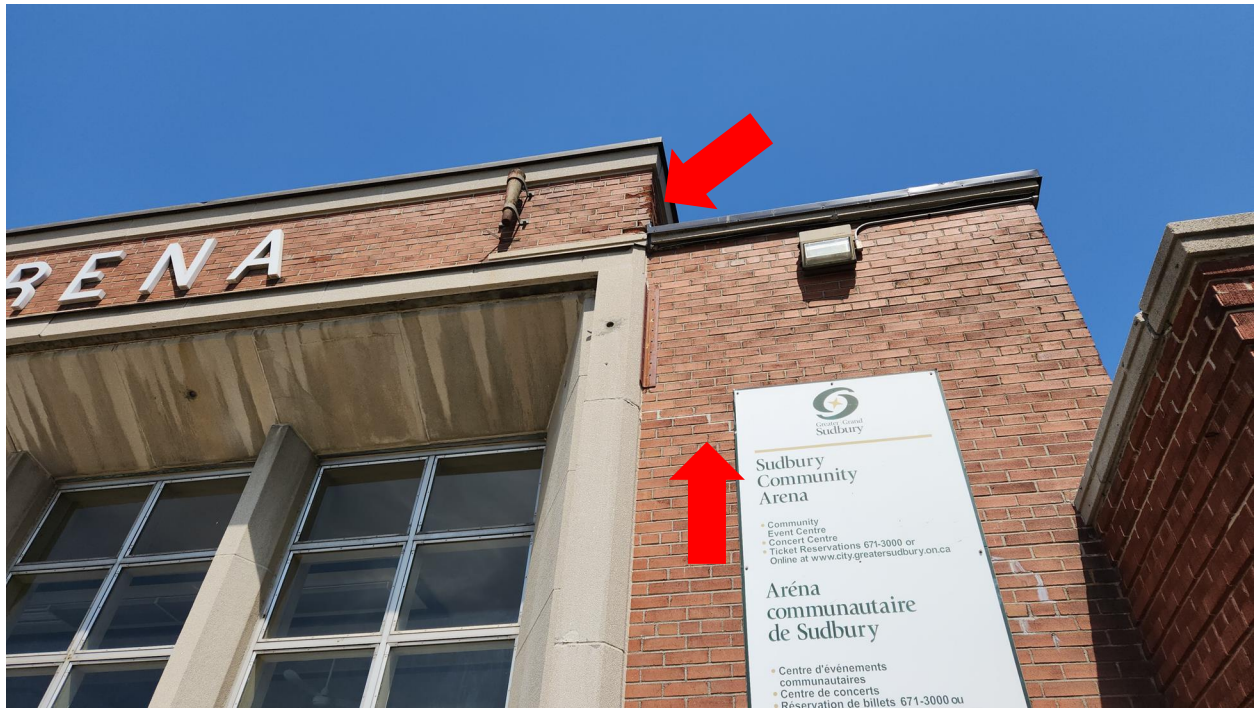
Photo 31: Damaged and cracked brick masonry (c.1951).
