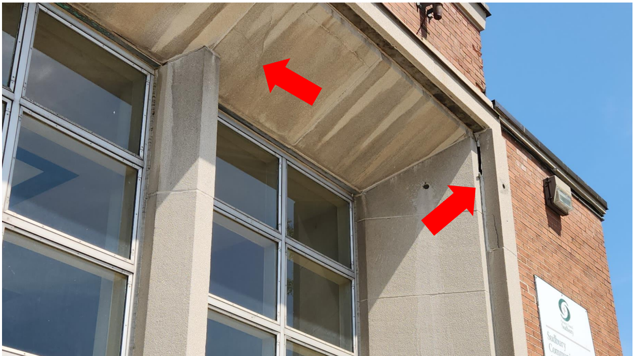
Photo 36: Cracked precast concrete at Main Entrance (c.1951).
