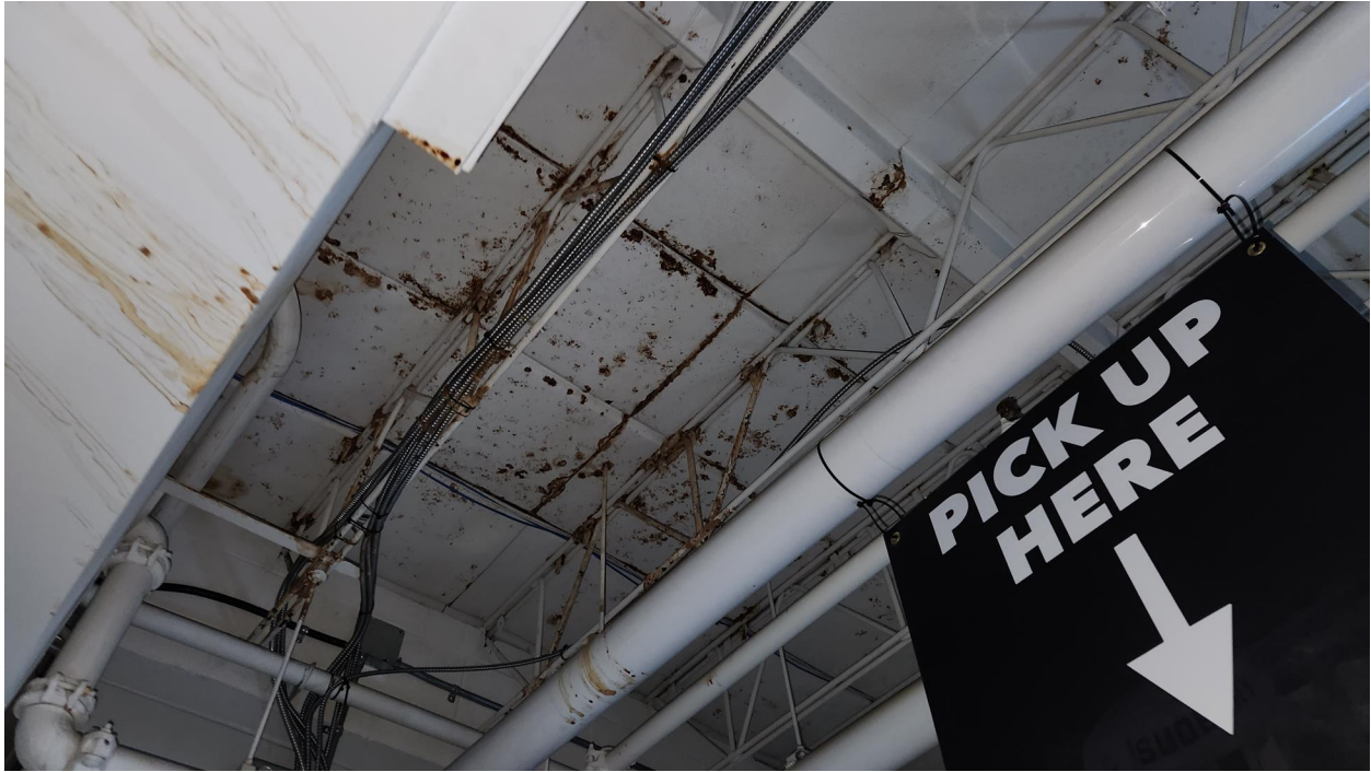
Photo 7: Deterioration of Low Roof structure at northwest corner (c.1951).
