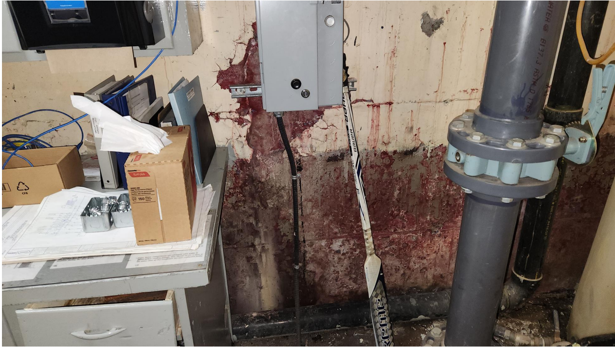
Photo 15: Evidence of leakage through concrete foundation wall in the Mechanical Room (c.1951).
