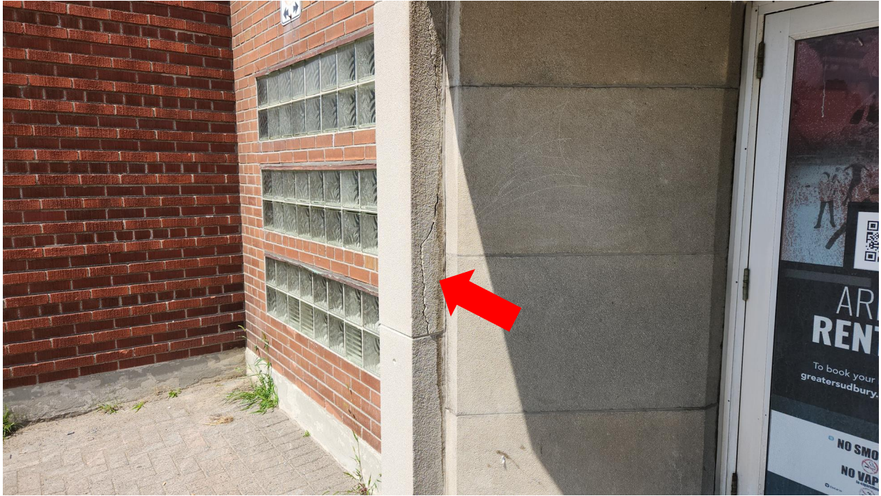
Photo 35: Cracked precast concrete at Main Entrance (c.1951).
